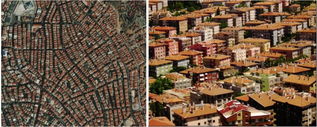
Figure 5.3. Yücel-Uybadin Plan shaped by the development of the Küçükkesat neighborhood islands (left) and the typology of the housing produced in the relevant period (right) – (Source: Bing Satellite Image, 2019; Çalışkan’s personal archive, 2004)
