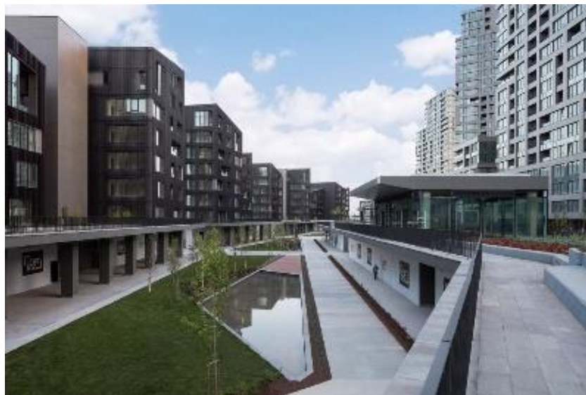
Figure 5.16. Incek Loft's 'platform' and 'section' image - (Source: Incek Loft Official Web Page, 2018)
