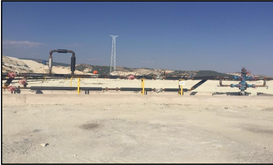
Figure 23. Wellhead of production well
