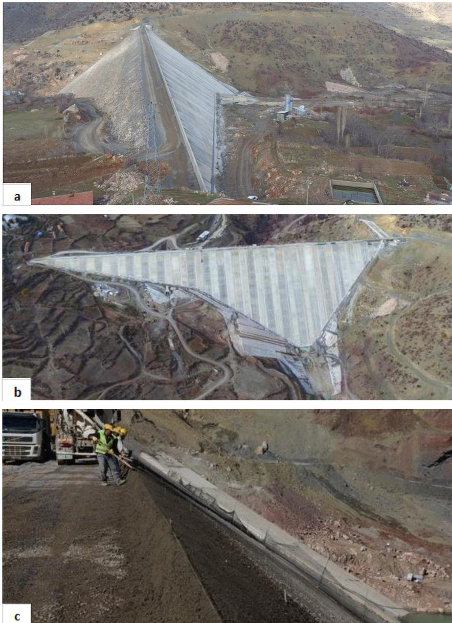
*Figure 3.4. a) Longitudinal South and b) Upstream Top Views of Afşar Dam, c) Embankment Construction*
