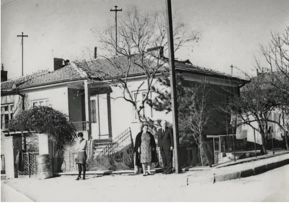
Figure 3.6. A Residential Unit in Yenimahalle from 1960s. Şinasi Yüksel's Individual Archive. Retrieved from http://www.sinasiyukse.com/blog/?p=17727 .
