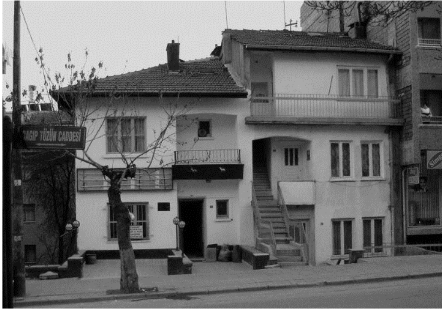
Figure 3.8. A residential Unit in Yenimahalle from 1960s. Şinasi Yüksel's Individual Archive. Retrieved from http://www.sinasiyüksel.com/blog/?p=17727 .
