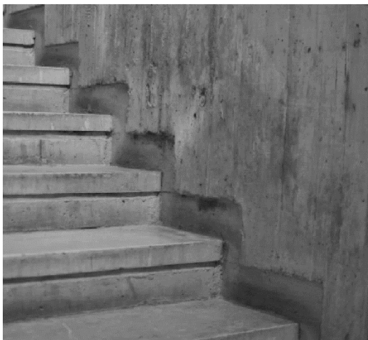
Figure 25: Skirting board gaps from the Faculty building.
