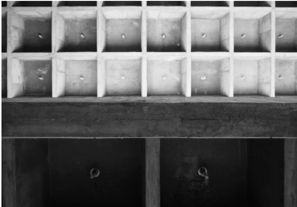
Figure 54: Waffle slab structure of the METU Faculty of Architecture building
