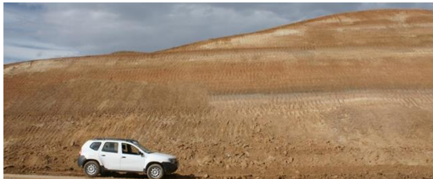
Figure 5.106. General view of KM:107+100 cut slope
