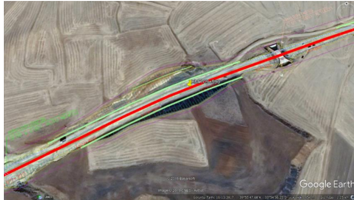
Figure 4.2. Google Earth view of KM:109+590 cut slope
