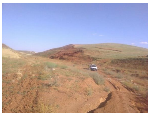
Figure 4.5: General view of KM:113+120 cut slope
