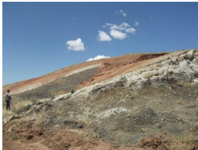
Figure 4.3. General view of KM:109+590 cut slope
