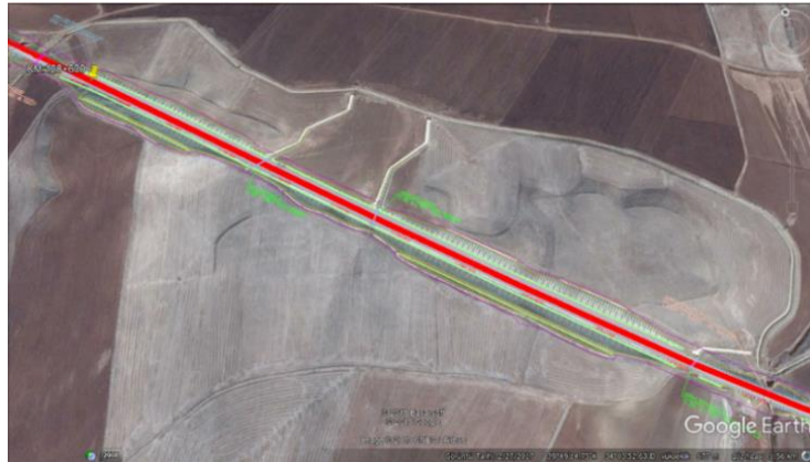
Figure 4.9. Google Earth view of KM:128+630 cut slope
