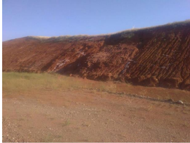
Figure 4.8: General view of KM:121+200 cut slope
