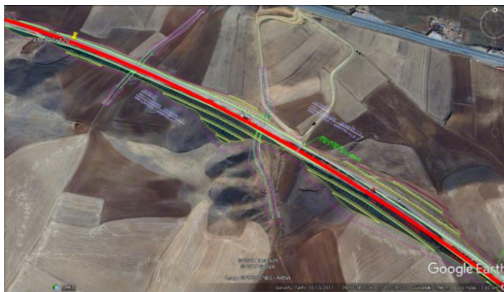
Figure 4.4. Google Earth view of KM:113+120 cut slope
