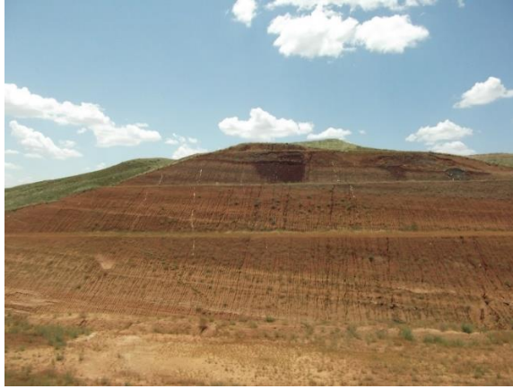
Figure 4.6. Seepage of surface waters and rill erosion on KM:113+120 cut slope
