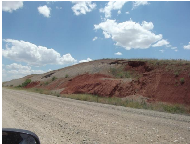
Figure 4.10: General view of KM:128+630 cut slope
