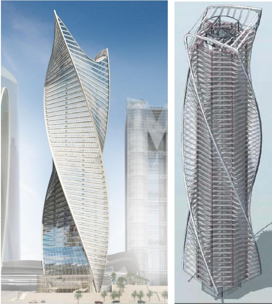
Figure 2.19: Evolution Tower and 3D model of structural members. (Nikandrov, 2016)
