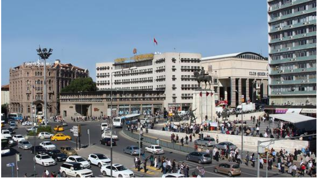
Figure 4.9. Ulus Square General View From South West 4 . (Çalık, 2019 January)
