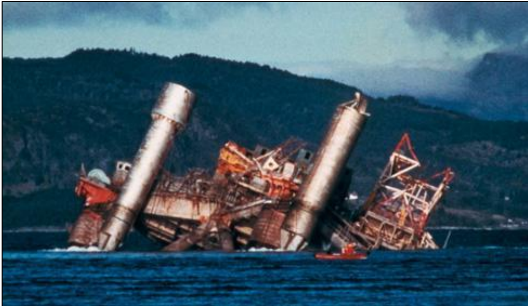
Figure 1-5: North Sea Alexander L. Kielland Oil Rig Collapse, [13]
