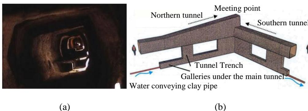
Figure 2.1. The Tunnel of Samos (a) Cross Section of the tunnel (Apostol, 2004); (b) A sketch of meeting points of the tunnel boring sections (Angistalis and Kouroumli, 2014)
