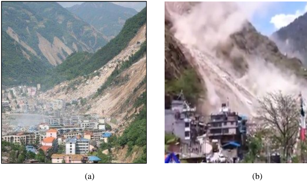
Figure 1.1 (a) Earthquake-induced slope failure of a natural slope in 2008 Wenchuan Earthquake (source: sciencedaily.com), (b) failure of a natural slope after the 2015 Nepal-Gorkha Earthquake caught on camera ((source: indianexpress.com)
