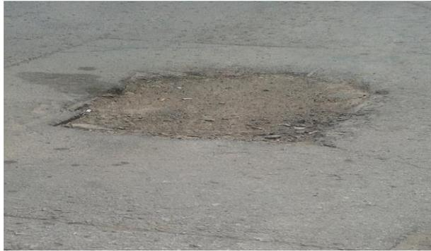
*Figure 3.1. A pothole with STD < 10*
