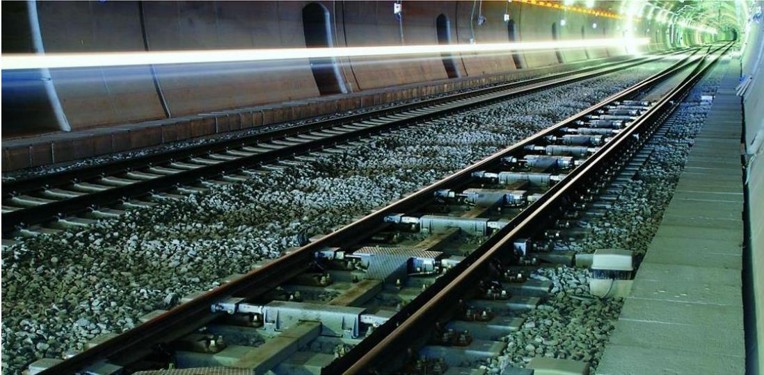
**Figure 35** Hy-Drive point machine solution installed on a multiple drive turnout [24]
