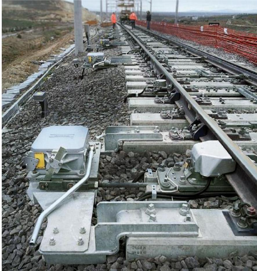
**Figure 29** Multiple drive integrated into high speed line turnout in Turkey [19]
