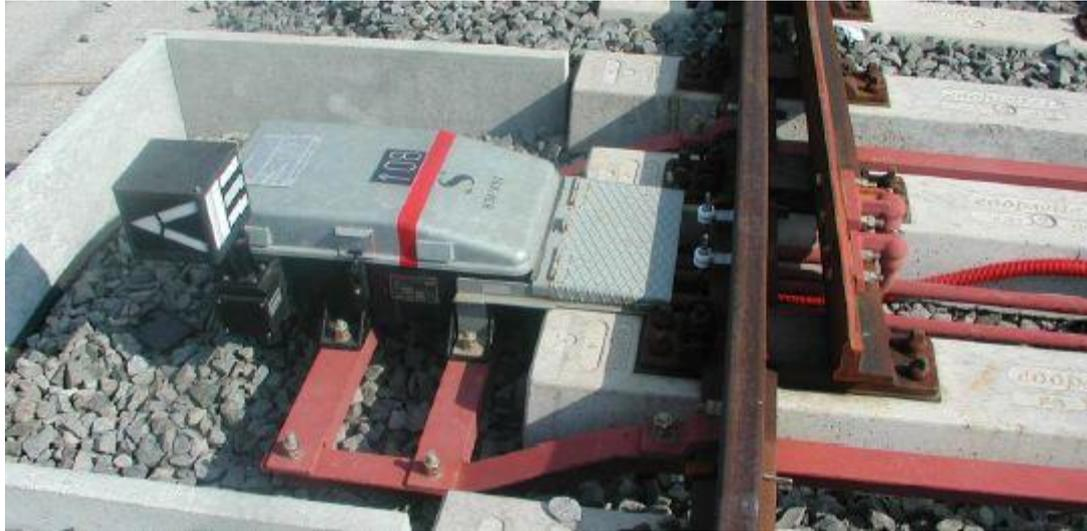
**Figure 34** The photograph of P80 point machine installed near the track [23]
