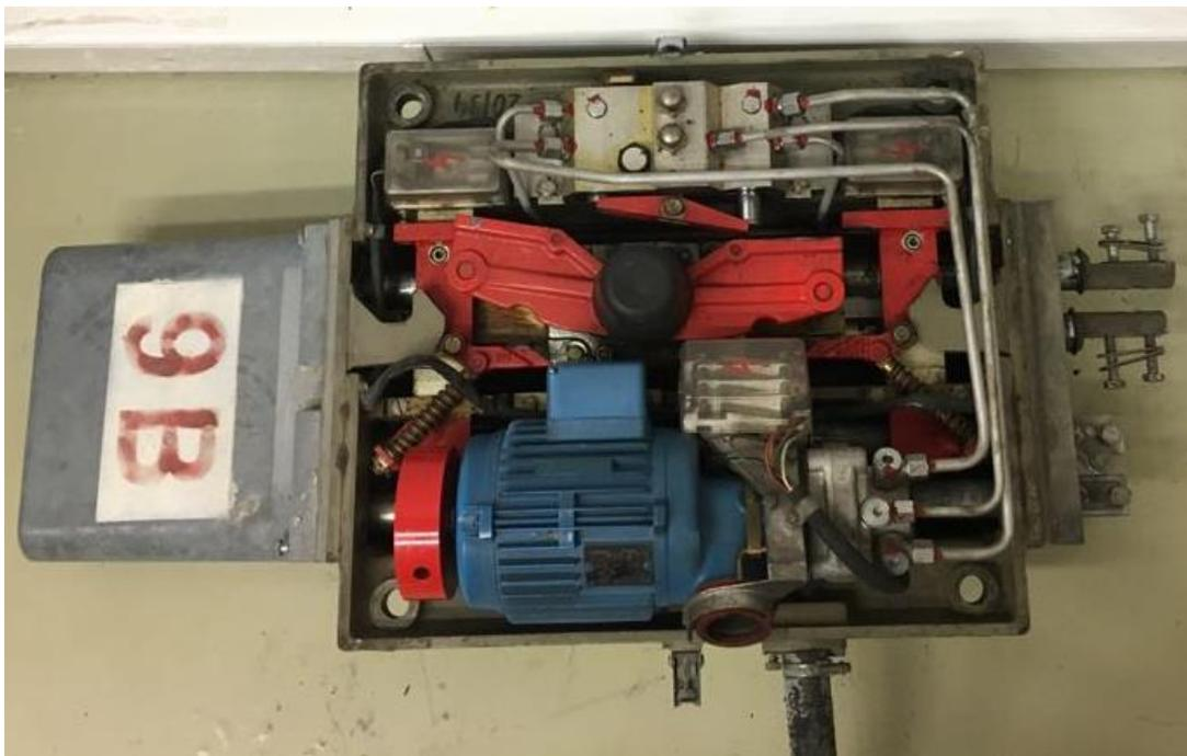
**Figure 83** Photograph of inside view of point machine C
