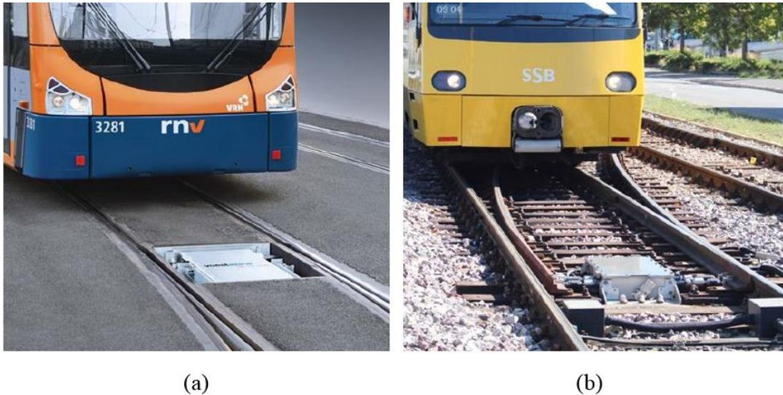
**Figure 20** Unistar CSV 24 point machine embedded track, 1000 mm track gauge (a) and open track, 1435 mm track gauge (b) [16]
