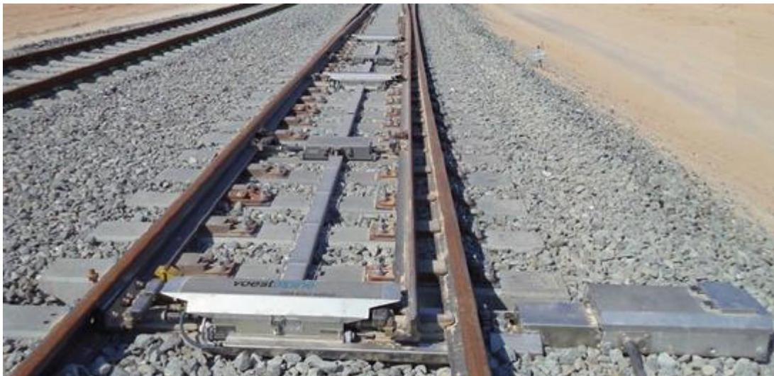
**Figure 22** Unistar ELP modules installed between DLD modules [17]
