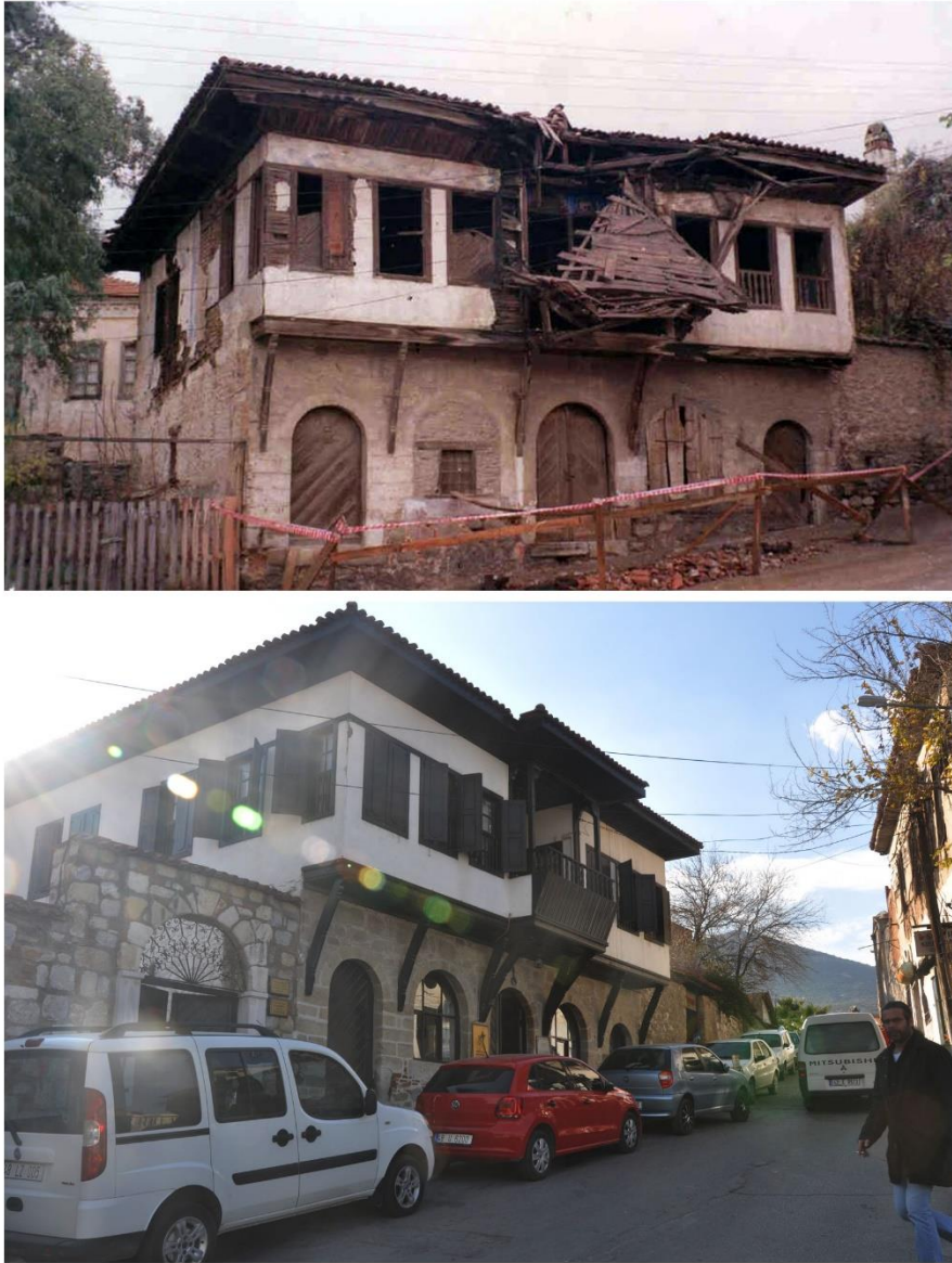
Figure 4.73. The Mansion of Hacı Ali Ağa before the restoration (top) (Milas Municipality archive), after the restoration (bottom) (Author, Dec, 2016).
