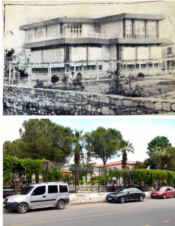
Figure 4.26. Milas Museum and Public Library as new constructed (top) (Olçay Akdeniz personal archive), (bottom) (Author, May, 2017).
