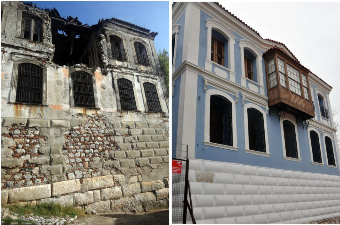
Figure 4.83. The Mansion of Emin Ağa before the restoration (left) (Güliz Bilgin Altınöz personal archive), after the restoration (right) (Author, Dec, 2016).
