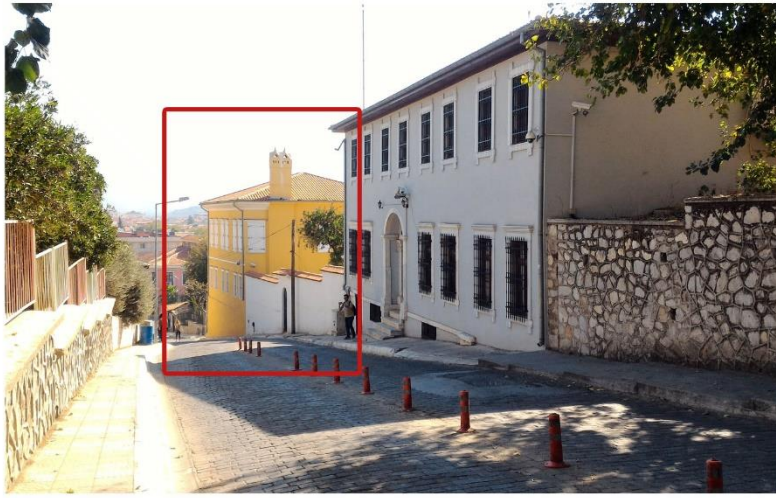
Figure 4.76. The building before the excavation (top) (Uzunyuva Expropriation Report), after the restoration (bottom) (Author, Oct, 2017).
