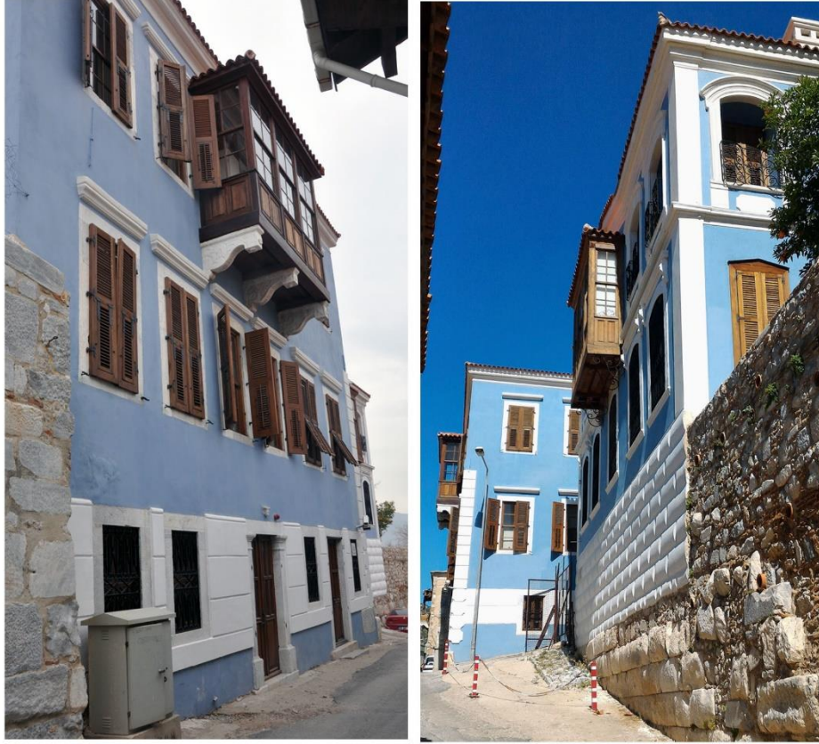
Figure 4.12. Kolağası/ Çorbacı Mansion (left) (author, Dec, 2016), Kolağası Mansion and Emin Ağa Mansion (right) (author, May, 2017).
