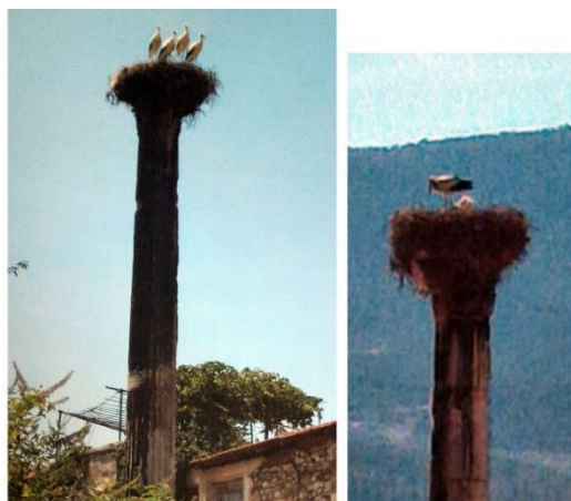
Figure 4.3. Uzunyuva Column as the “nest of storks” (left) (Akdeniz, 2010), (right) (Author, May, 2017)
