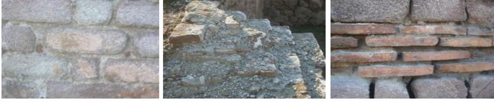
**Figure 3.24** Mortar examples in the Bath
