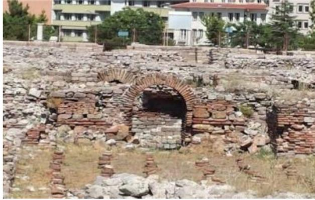
**Figure 3.22** The brickwork of arches and *pilae* (photo: Zeynep Tanrıverdi, 2014)
