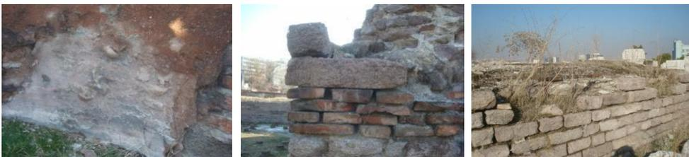
**Figure 3.26** Material lost, efflorescence and biological growth on materials of the Bath (photos: Zeynep Tanrıverdi, 2014)
