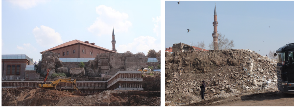
Figure 72 The demolition in Sub-Area 2 for the construction of underground carpark Source: A. Güliz Bilgin Altınöz Archive
