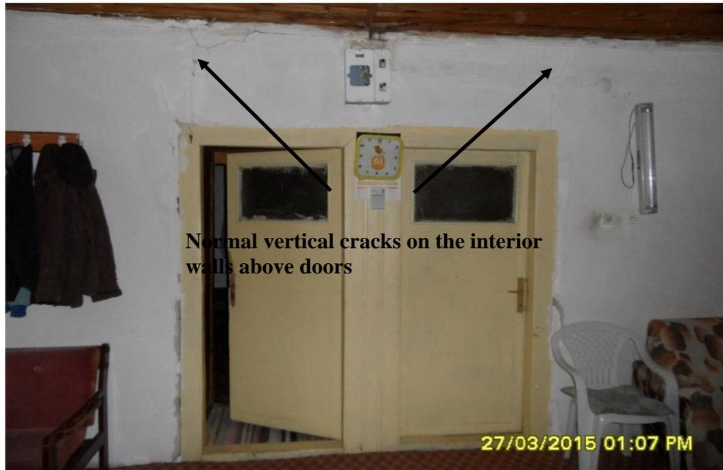
Figure 4.9 Normal vertical tension cracks above the door corners in the first floor of Sami Yıldırım's house (Bilgin et al., 2015)
