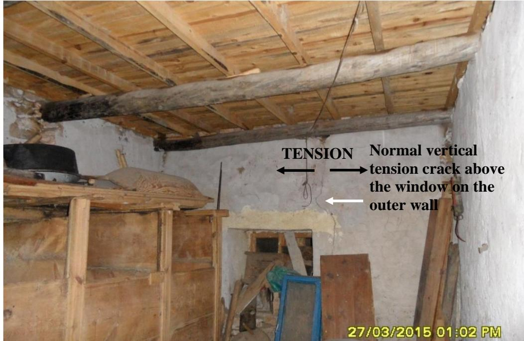
Figure 4.10 Normal vertical tension crack above the window in the basement of Sami Yıldırım's house (Bilgin et al., 2015)
