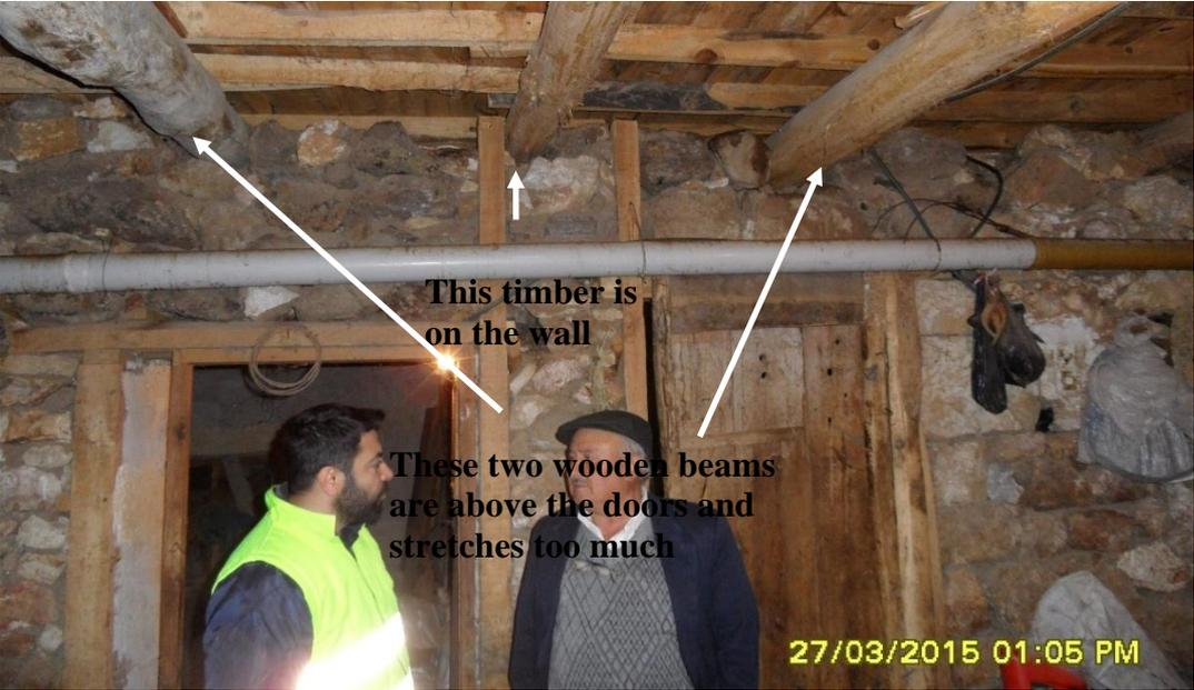
Figure 4.8 Mud-mortared walls and wooden beams in the basement of Sami Yıldırım's house (Bilgin et al., 2015)
