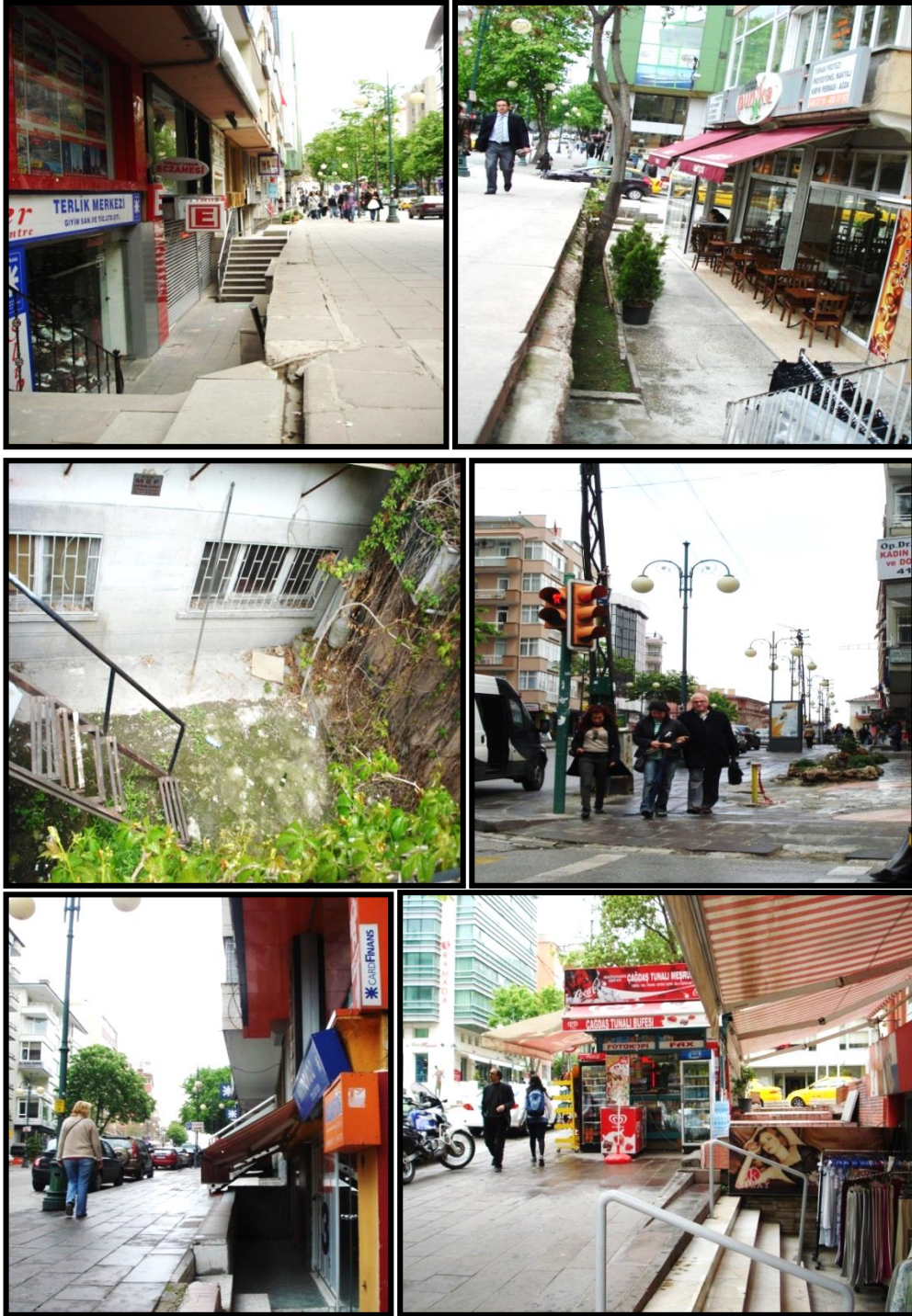
Figure 6.35, Unsafe level variations on the sidewalk of THS (Re: Personal archive)
