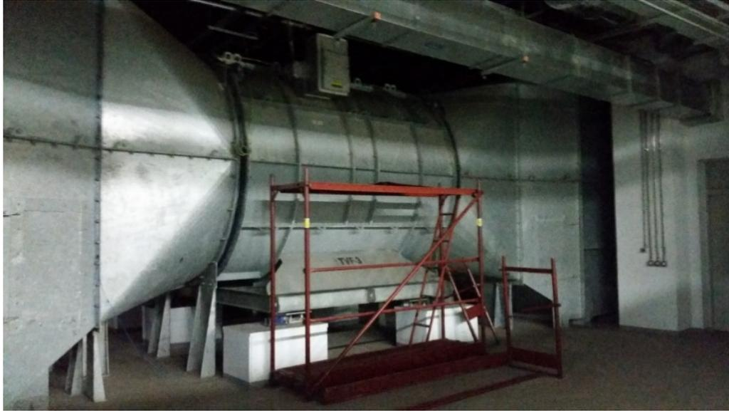
Figure 1.12: Marmaray Tunnel ventilation fan
