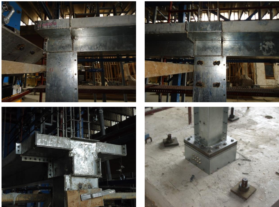
Figure 3.4 Assembled formworks
