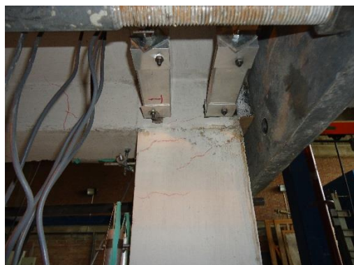
First story exterior column top end
