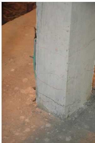
First story interior column bottom end
