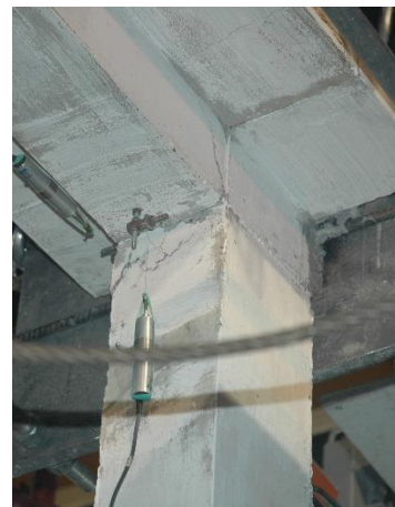
Second story exterior column top end
