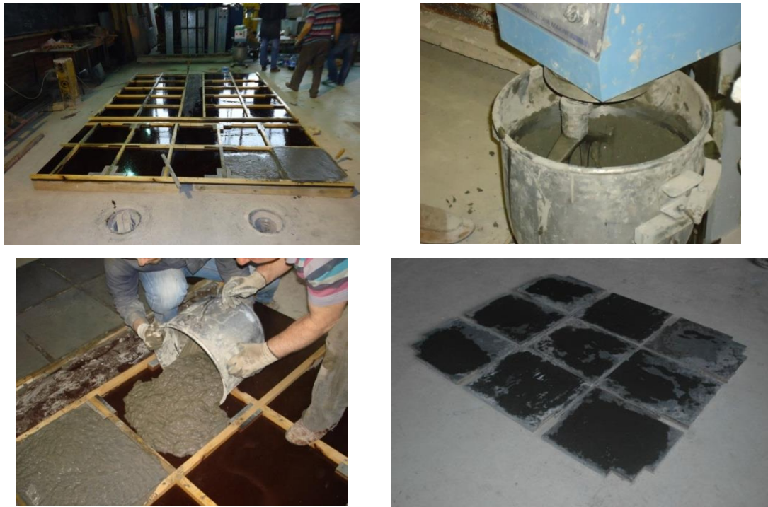
Figure 2.5 Production of ECC panels
