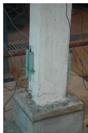
First story exterior column bottom end
