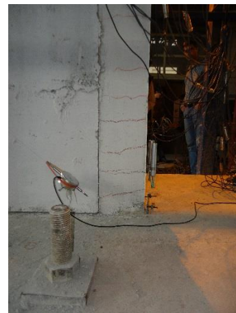
First story interior column bottom end
