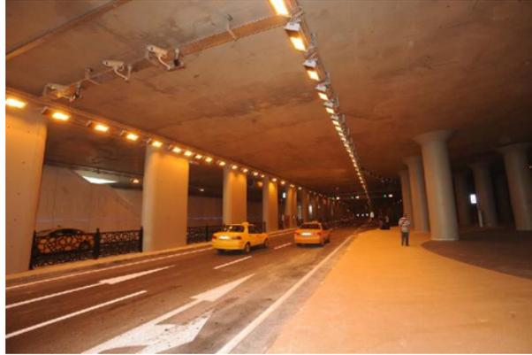
Figure 2.19: The Lighting and Camera System in Taksim Square Tunnel, Istanbul [8]
