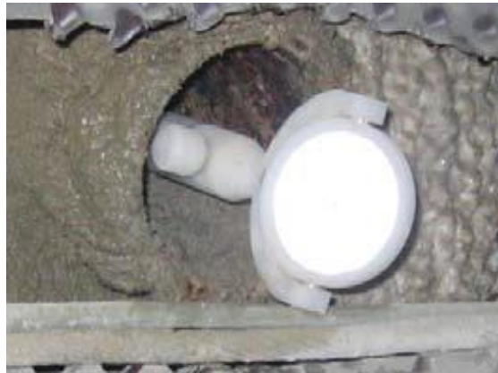
Figure 4 Monitoring Target with Protection Pipe
