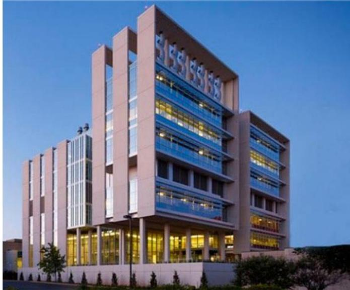
Figure 13: Oklahoma Medical Research Foundation building. The flow is channeled to wind turbines by planes designed on roof. Source: <http://perkinswill.com/work/oklahoma-medical-research-foundation.html>, accessed at 15.03.2016
