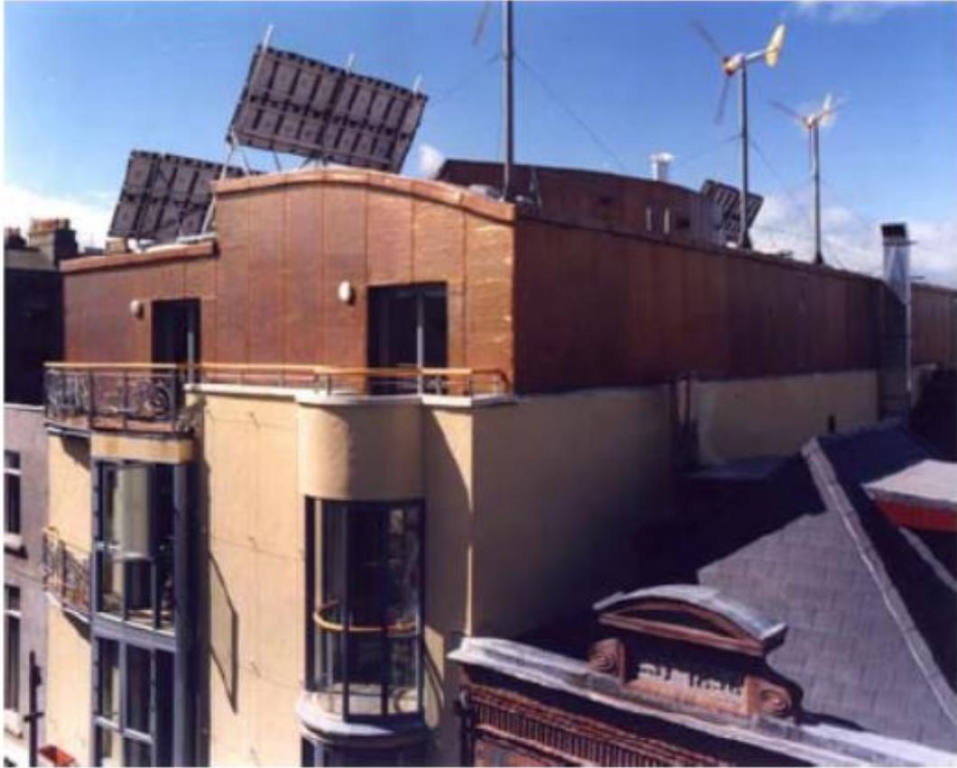
Figure 9: Green Building, Temple Bar, Dublin, 1995. Three turbines (each 1,5 kW) developed by Murray O’Laioire Associates (Dutton et al., 2005)
