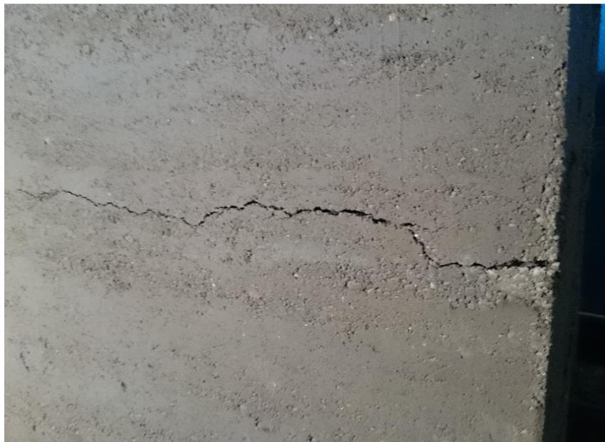
Figure 3.42 Cracks because of shrinkage
