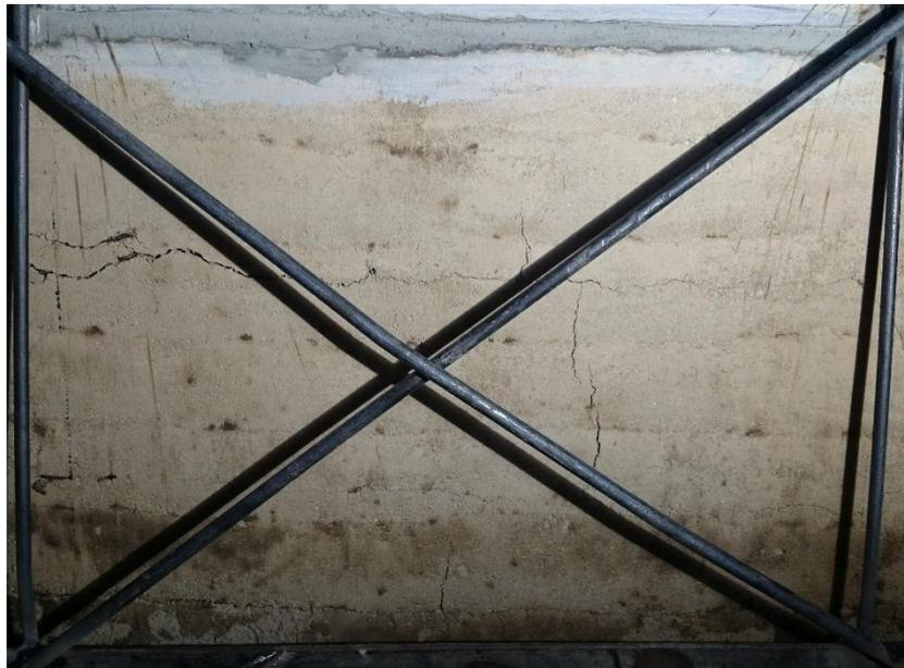
Figure 3.45 Addition of vertical + diagonal reinforcements
