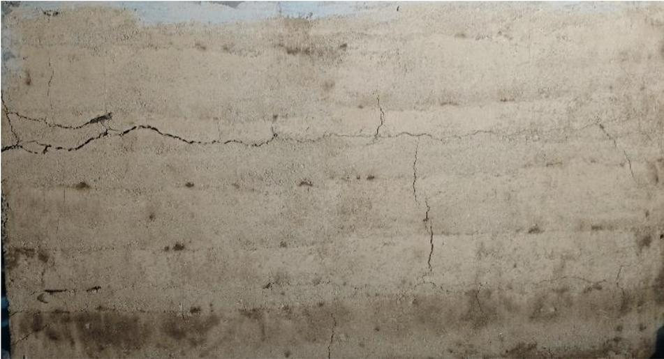
Figure 3.43 Shrinkage cracks after curing
