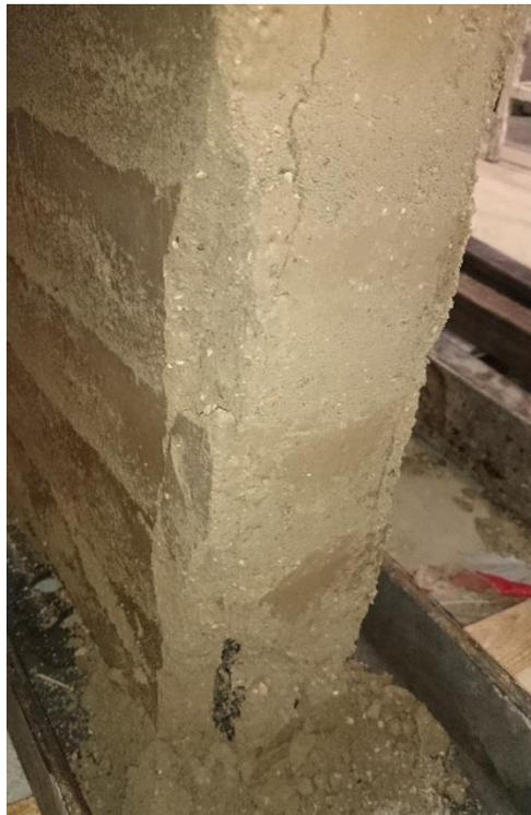
Figure 3.33 Cracks at the sides
