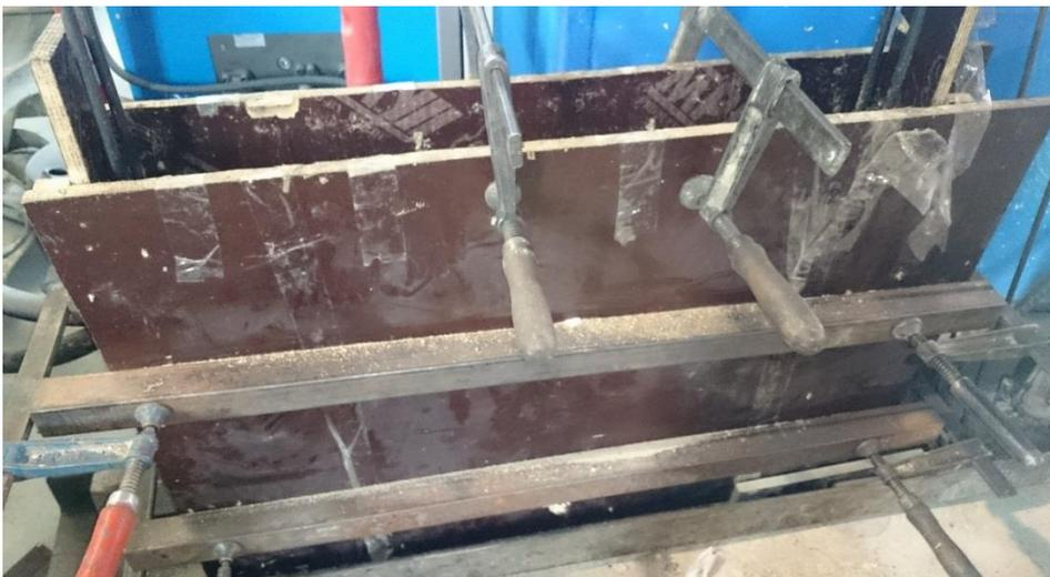
Figure 2.28 Formworks with supports
