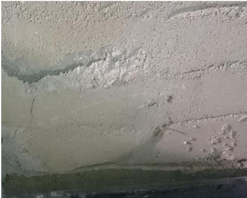
Figure 3.30 Expansion of the cracks at joint
