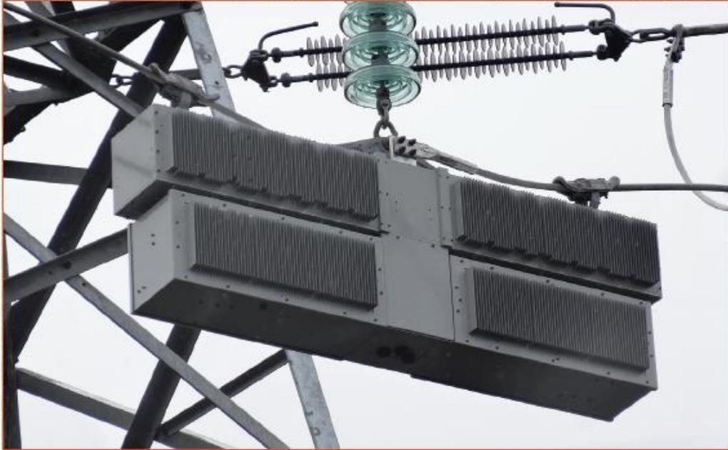
*Figure 3 Installed DSSC [10]*
