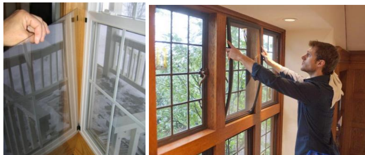
Figure C.13. Storm window panels; left: clear acrylic plastic sheet; right: flexible inside storm panel. ( http://www.builditsolar.com and http://green-conscience.com , respectively).
