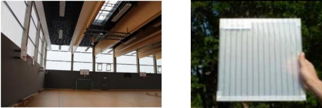
Figure C.3. Example of granular aerogel filled PC panels (Moretti, et al., 2017).
