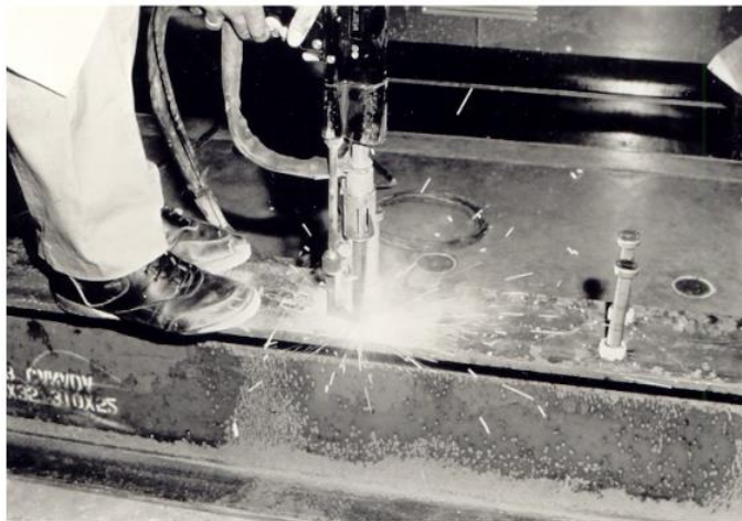
Figure 1.8. Welding of stud shear connector using a welding gun (Pashan, 2006)
