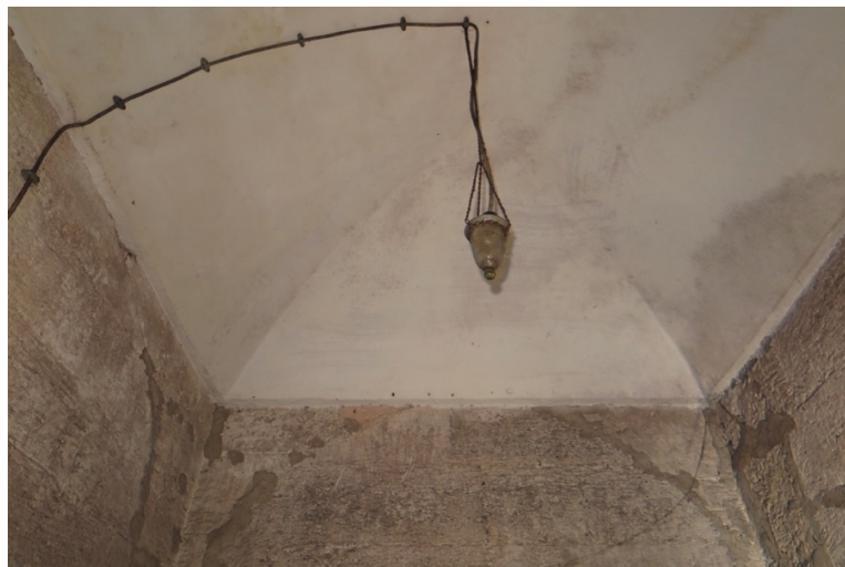
Figure 150: The cloister vault covering the space over the staircase leading to the mahfil floor (by the author, 2015)
