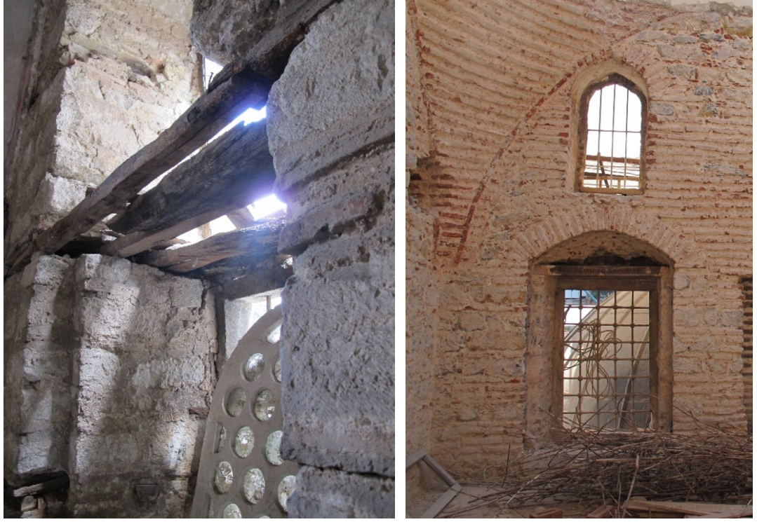
Figure 52: Use of timber lintels for the window openings with relieving arches in the Atik Valide Darülcürri and Medrese (by the author, 2014)
