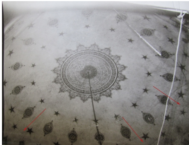
Figure 142: The circular plaster cracks which may indicate the level of the tension ring (VGM Archive, 1982)
