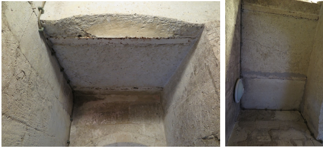
Figure 133: The stone slabs which are supported by auxiliary iron beams (by the author, 2016)
