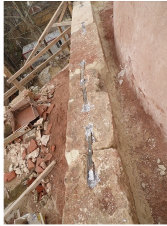
Figure 144: The top surface of the drum of the Lüleburgaz Sokullu Mehmed Paşa Hamam 's dome during the restoration process. Photograph showing the clamps some of which were changed with new ones. (Lüleburgaz Municipality Archive, 2013)
