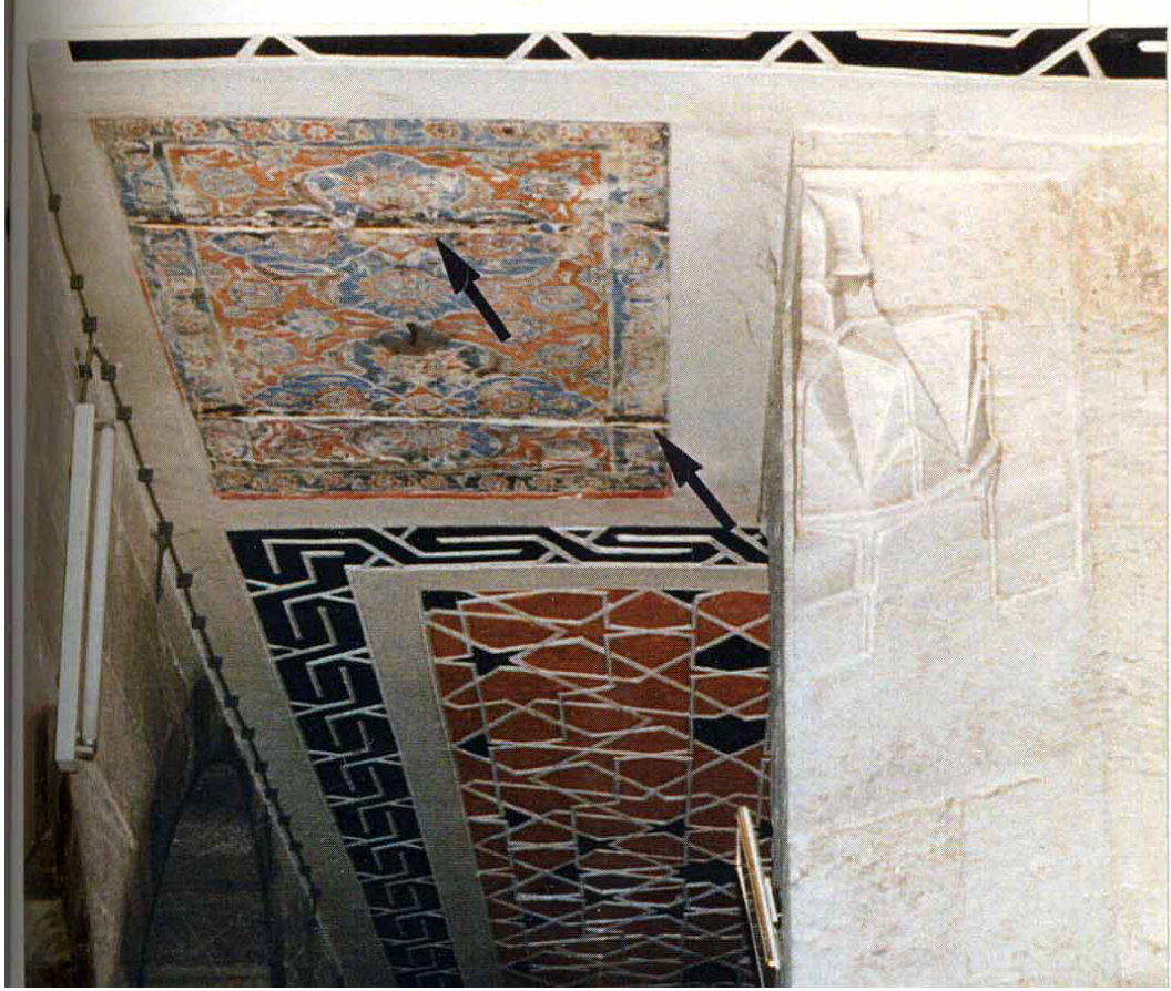
Figure 35: The auxiliary iron beams supporting the slab of the mahfil ( (Tanyeli G. , 1990, p. 236)
