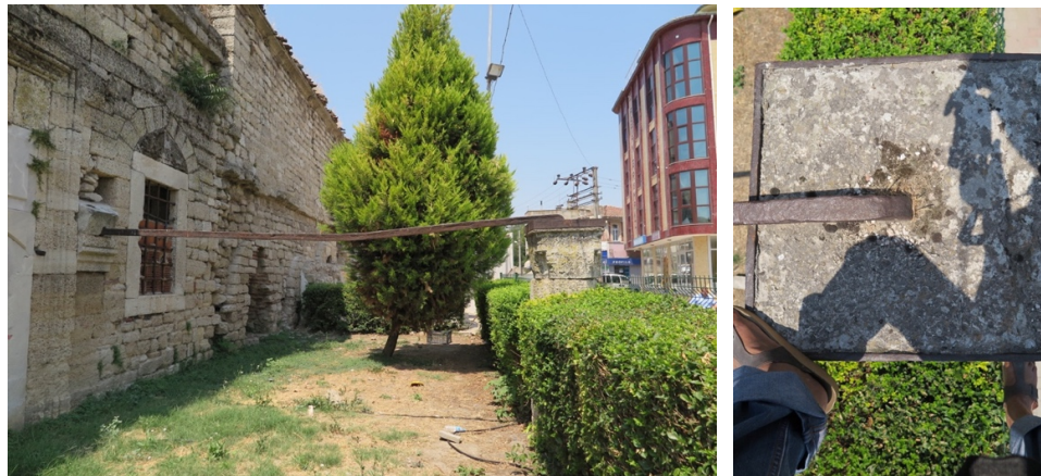
Figure 122: The iron tie bar of the Havsa Sokullu Mehmed Paşa Hamam 's arcade (By the author, 2015)
