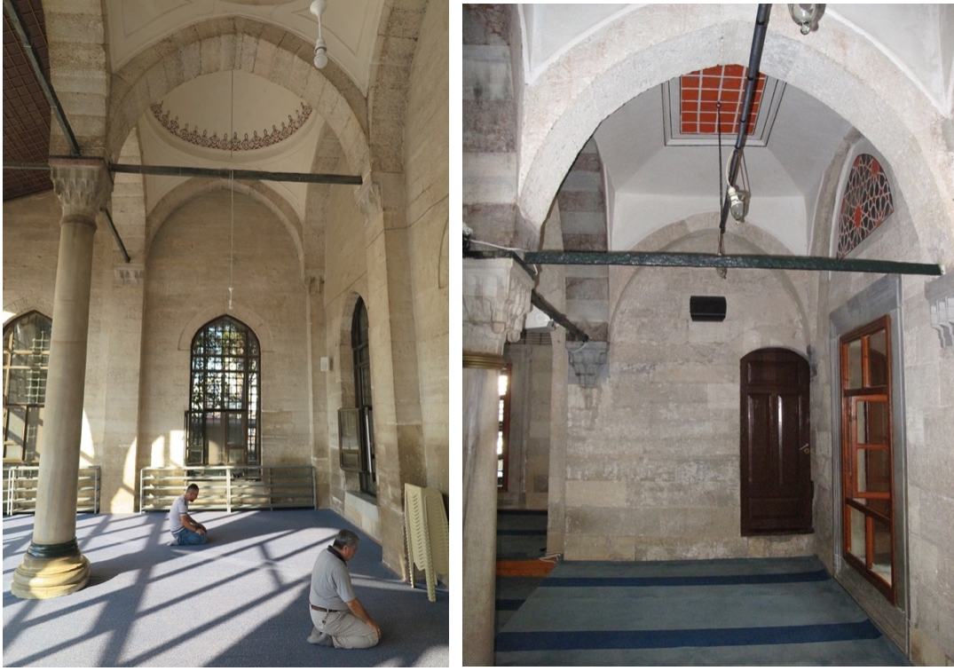
Figure 124: Arches of type 2. The photo on the left is from the last prayer hall (by the author, 2015). The photo on the right is from the yan sahn on the east side (by the author, 2014)
