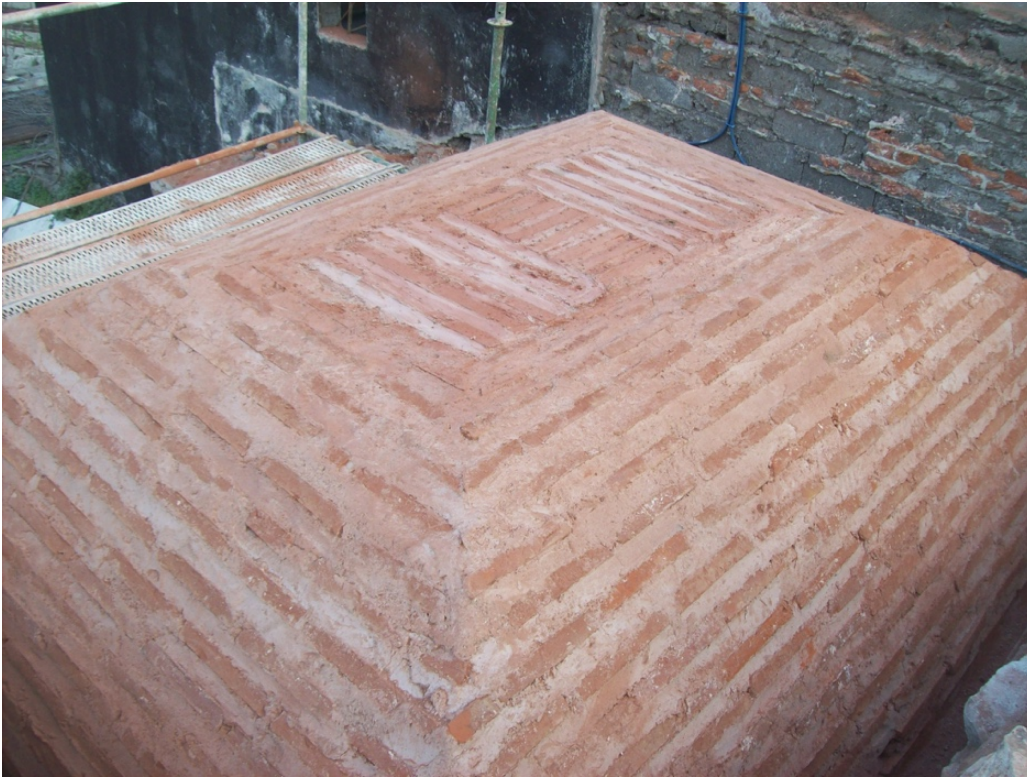
Figure 151: The reconstruction process of the vault with shouldered profile in Süleymaniye Rabi Medresesi by using traditional materials and techniques (Archive of Sayka Construction and Architecture, 2008)
