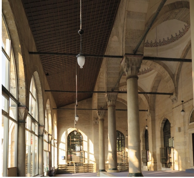
Figure 153: The timber roofing of the second arcade of the last prayer hall (by the author, 2016)
