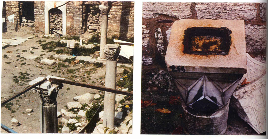
Figure 38: (Left) The tie surrounding the arcade of Davut Paşa Medrese and the iron ring of the column capital in the Topkapı Palace Kitchen's garden ( Tanyeli G. , 1990, p. 245)
