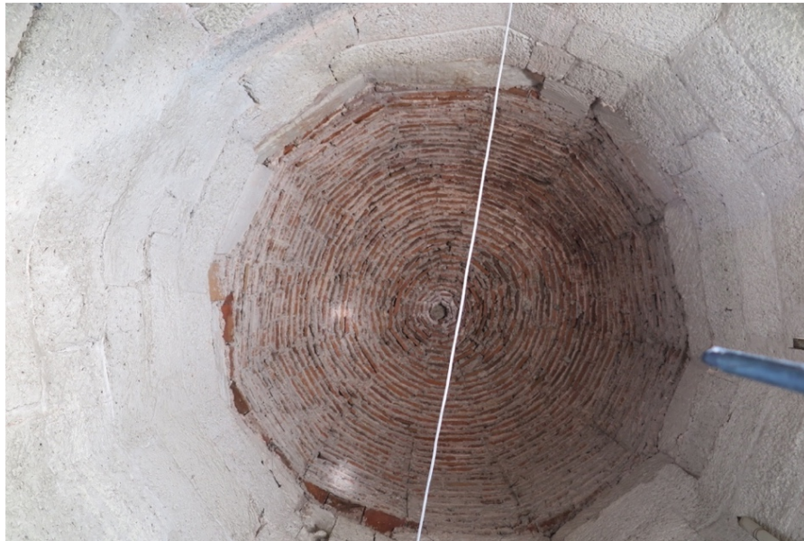
Figure 148: The domical vault covering the weight tower at the north-west corner (by the author, 2015)
