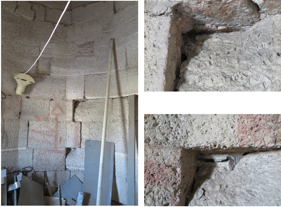
Figure 118: The wall of the weight tower fastened by iron clamps (By the author, 2015)
