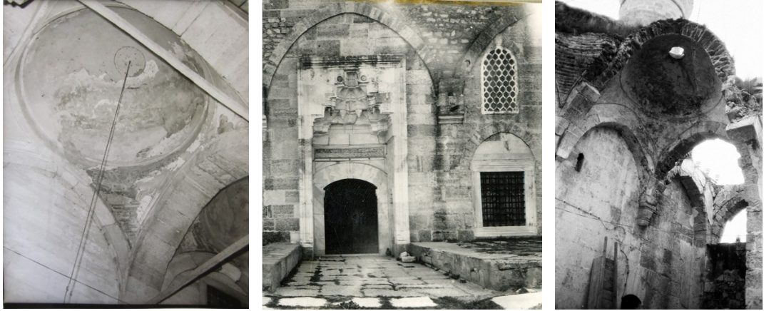
Figure 140: (Left) The pendentive and the dome of the last prayer hall in Lüleburgaz Sokullu Mehmed Paşa Mosque (VGM Archive, 1950s); (Mid) The back fill of the pendentive of Havsa case (VGM Archive, 1980s); (Right) Demolished pendentive and dome of the last prayer hall in Payas case (VGM Archive, 1984).
