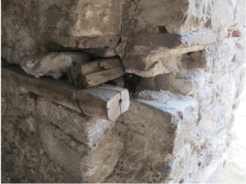
Figure 27: The photograph showing how the joint between a tie beam and a püştivan is. (by the author, 2014)
