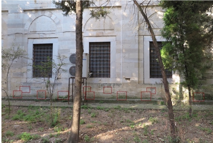
Figure 105: West Façade of the Lüleburgaz Sokullu Mehmed Paşa Mosque (By the author, 2015) The stone blocks, having nearly square shaped faces and located with similar intervals, can be also observed on east and south façades.
