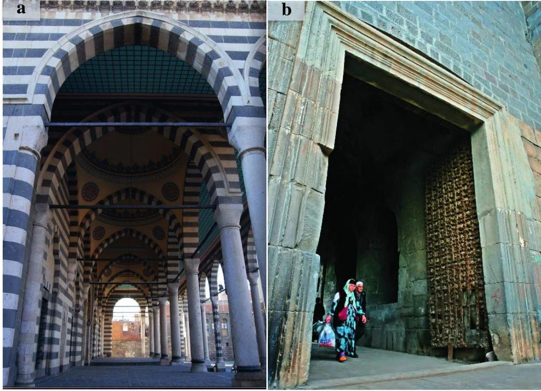
Figure 1.17 Limestone and metal applications (a) Alternation of limestone and basalt at Behram Pasha Mosque; (b) A metal door at Mardin Gate (Governorship of Diyarbakır, 2016)
