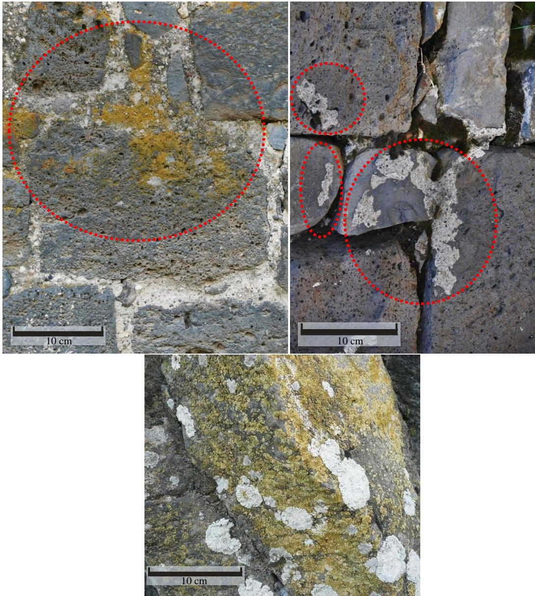
Figure 5.27 Lichens on sections of the DCW (lichens are indicated by dashed circles)
