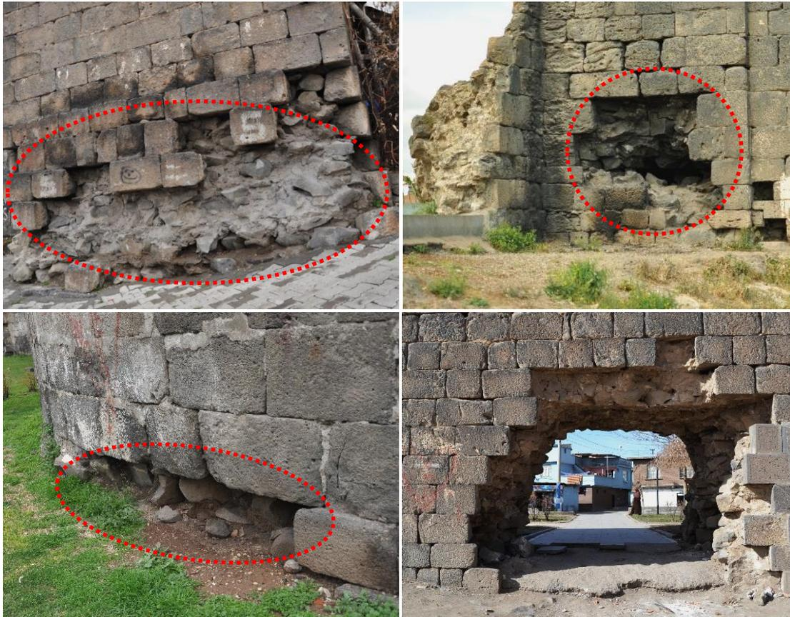
Figure 5.16. Dismantled stone blocks and a breach in the DCW (dismantled sections are indicated by dashed circles)
