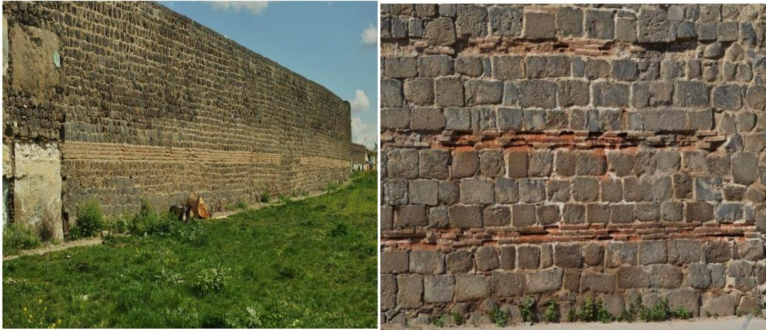
Figure 1.9 Opus listatum (east section of the DCW)
