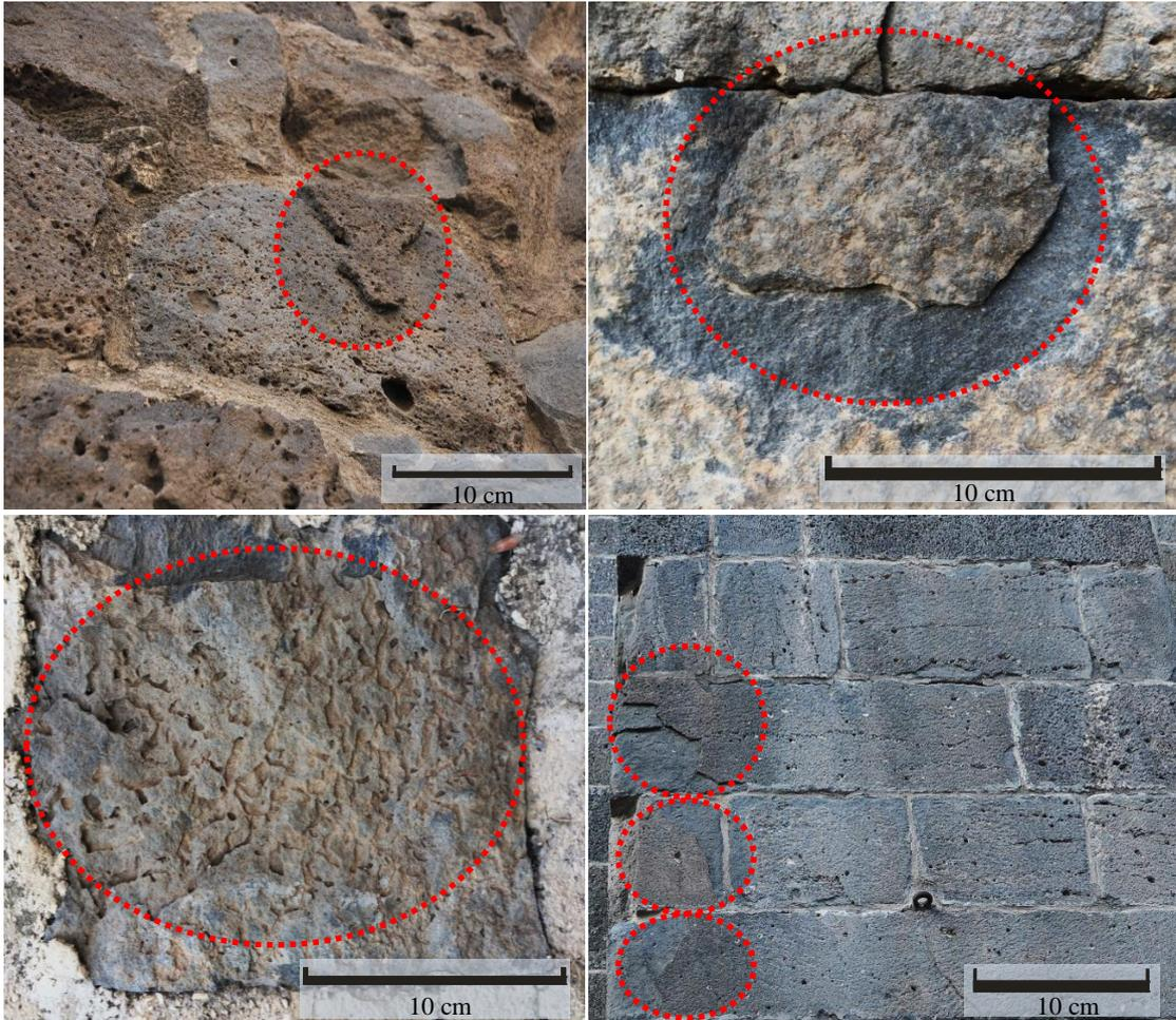
Figure 5.11 Scaling on sections of the DCW (scaling is indicated by dashed circles)
