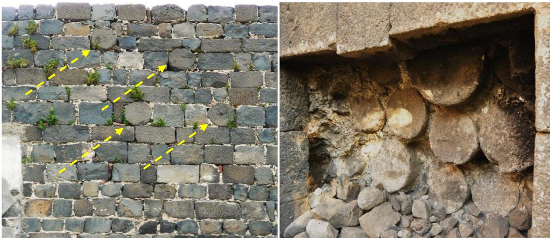
Figure 1.10 Cylindrical basalt applications (south and north section of the DCW)
