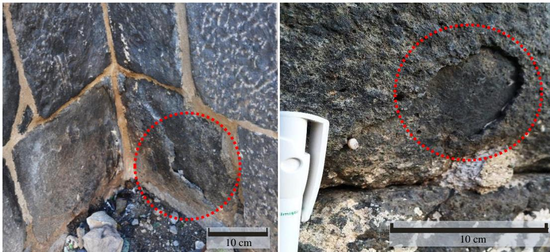
Figure 5.4 Blistering patterns at the lower parts of the walls (blistering patterns are indicated by dashed circles)
