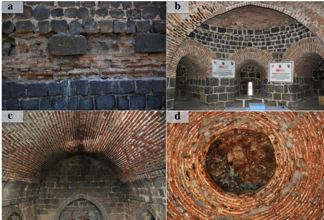
Figure 1.15 Brick applications on different sections of the DCW (a) Brick courses; (b) Brick domes and arches (Melikşah Tower); (c) Brick vault (Melikşah Tower); (d) Brick dome (Keçi Tower)
