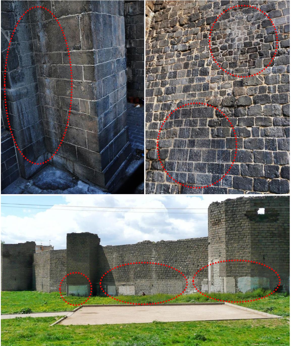
Figure 5.20 Deposits on the sections of the DCW (deposits are indicated by dashed circles)
