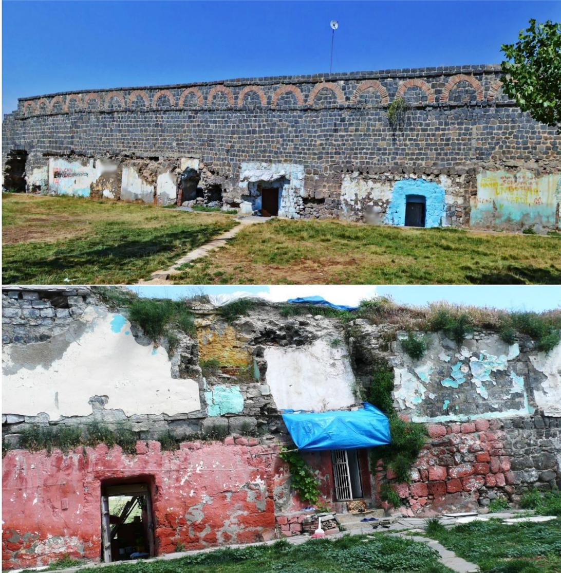
Figure 5.28 Paint and illegal housing on the east section of the DCW (the houses no longer exist, however, traces of them can be found on the walls)
