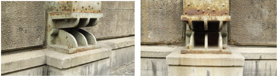
Figure 30. Part as a metaphor of function, pin-joints of Turbine Factory, Berlin, Peter Behrens. [Photographed by the author.]
