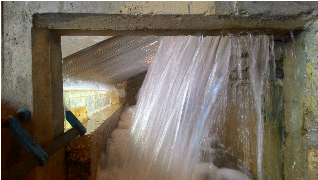
Figure 3.4 Trash rack and the sediment collection channel
