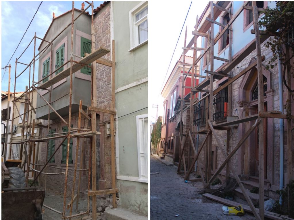
Figure 5.2 Examples for ongoing conservation projects
