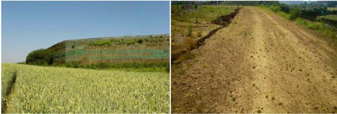
**Figure 2.3. A tensile crack behind reinforcement zone of a retaining wall which is made from reinforced soil (Vanicek, 2013)**
