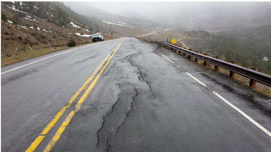
**Figure 2.2. Cracks on a highway surface which are caused by rainfall induced minor landslides on the highway embankment (Adopted from [www.codyenterprise.com](http://www.codyenterprise.com))**
