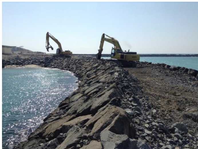
Figure 5.9 Breakwater built by rock
