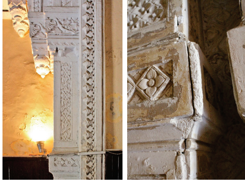
Figure 3.31: Gnd-N/02 – Entrance Vestibule – Deterioration (2016) Flaking paint on the Eastern Wall (Gnd-N/02-EW) (left), Flaked paint on and detachment of molded Plaster of Paris panels – (Gnd-N/02 EW) (right)
