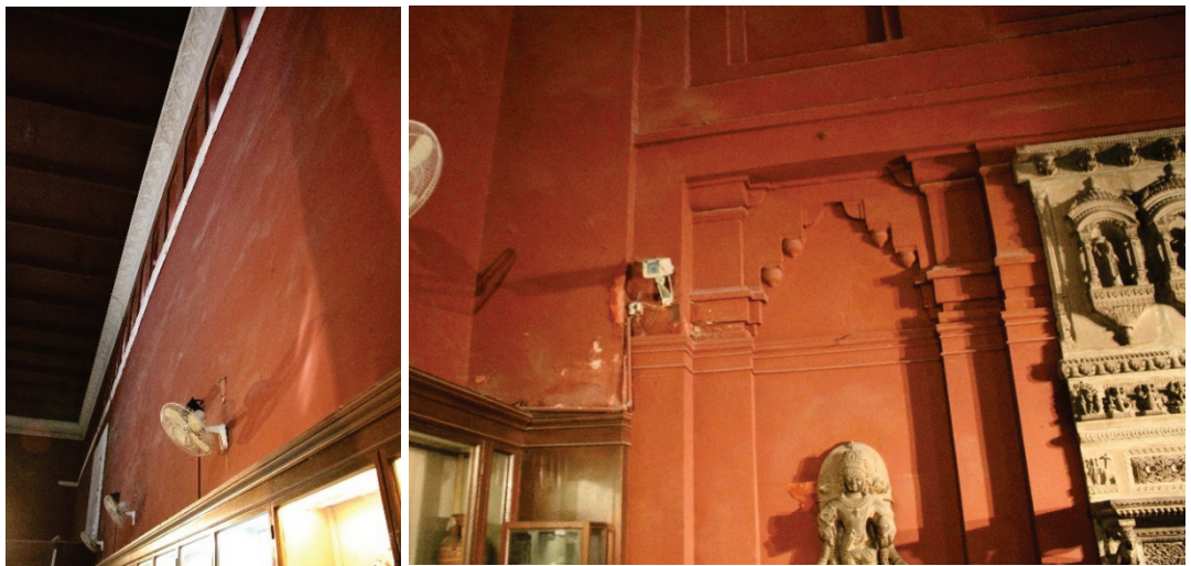
Figure 3.41: Gnd-E/03 – Hindu and Buddhist Gallery – Deterioration (2017) Plaster Swelling on Gnd-E/03-EW (left) and paint flaking on Gnd-E/03-SW (right)
