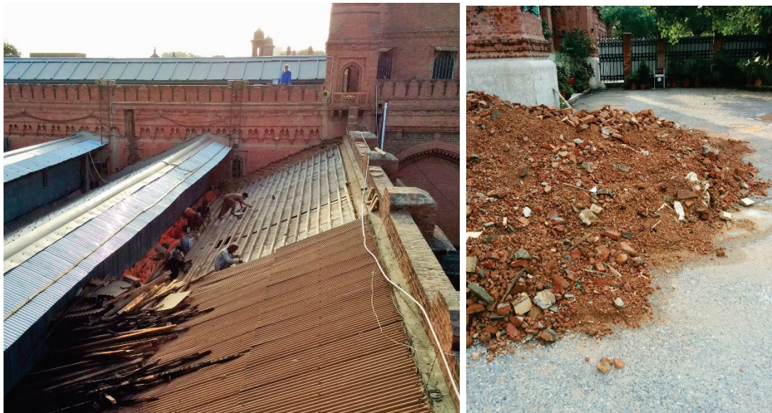
Figure 3.37: Gnd-E/01 – Islamic Arts Gallery – Roof Repairs (2015) Looking west over the roof (left), A pile of the lime concrete and brick tiles removed from the roof of the Islamic Gallery (Gnd-E/01) during repair works (right).
