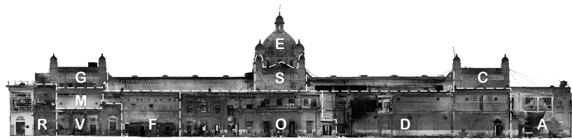
Figure 3.26: Lahore Museum– Southern Façade (2016) Orthographic projection from laser scan point-clouds. A: Laboratory, C/D/F/M/S: Galleries, E: Frontispiece, G: Auditorium and Library, R: Reserves Storage, V: Stores
