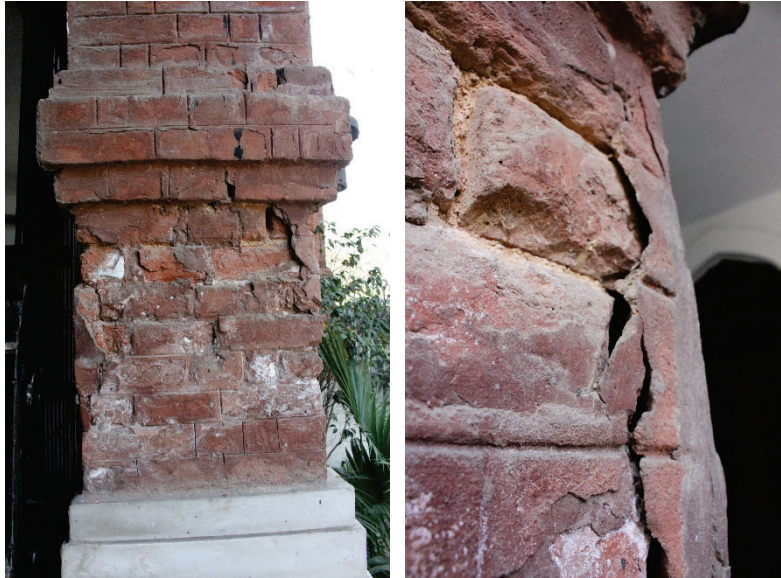
Figure 3.109: Gnd-W/09 – Auditorium & Library – Entrance Lobby (2016) Powdering and detachment of bricks
