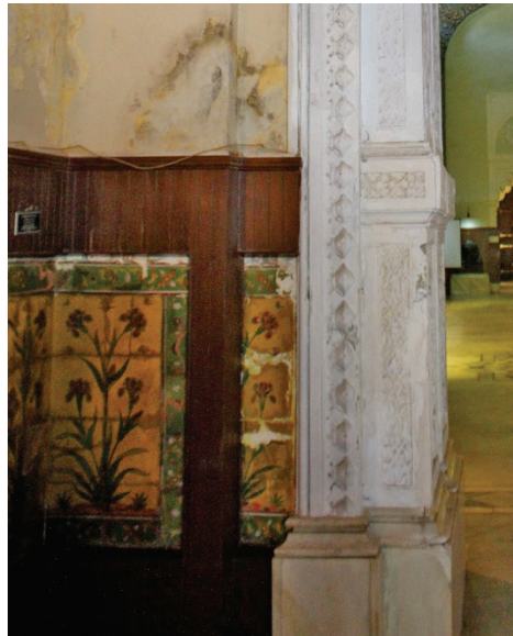
Figure 3.32: Gnd-N/02 – Entrance Vestibule – Deterioration (2016) Flaking of pain on the wall and efflorescence on glazed tiles – Southern Wall Gnd-N/02-EW
