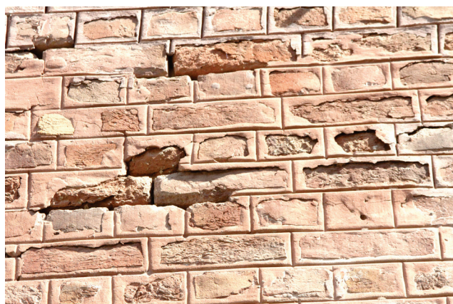
Figure 4.21: Fst-W/01 – Exterior Wall – Powdering of Brick / Detachment of Pointng (2017)
