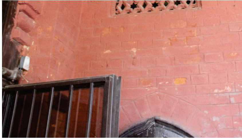
Figure 3.29: Gnd-N/01 – Entrance Portico (2016) Powdering of brick and flaking of the thin surface layer of red tinted cement.
