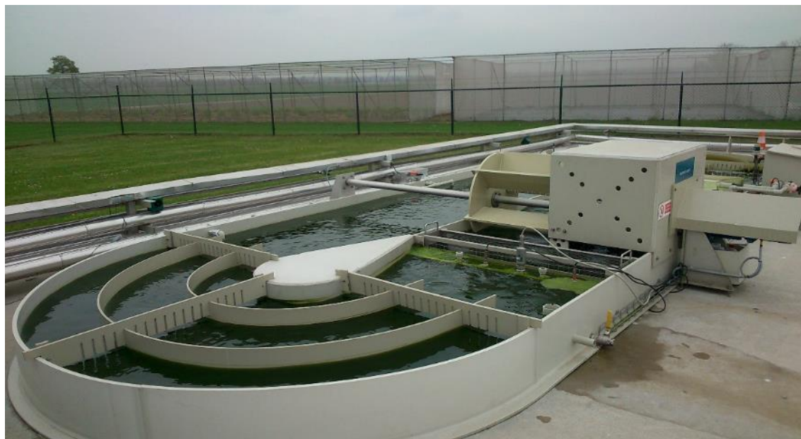
Figure 4 Photograph of a pilot scale raceway pond in AlgaePARC, Wageningen University, the Netherlands (Cakirlar, 2014)
