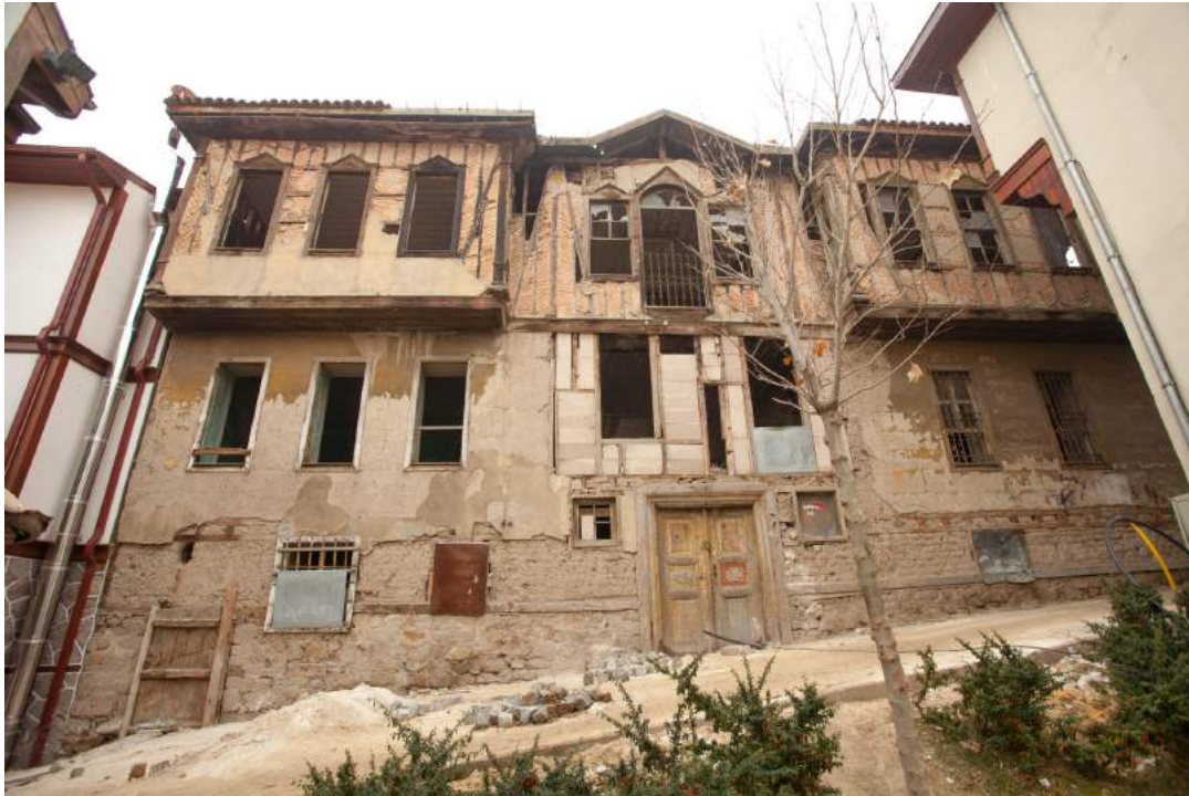
Figure 3.10: Block:19995, Lot:7; Traditional Technique, Timber Frame (RTT in Figure 3.8)
