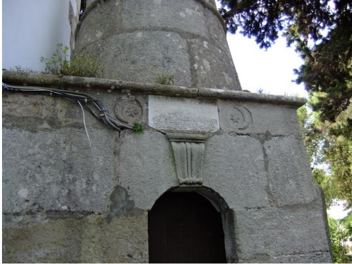
Figure 120 Entrance of the Cezayirli Ali Paşa Mosque's Minaret
