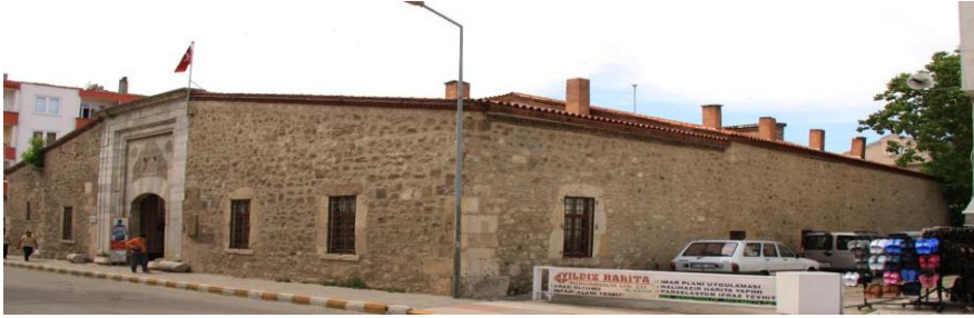
Figure 21 Pervane Madrasa from the Southeast
