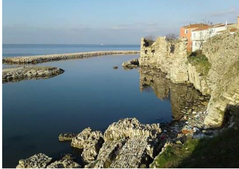
Figure 5 Northern Walls of the Sinop Citadel
