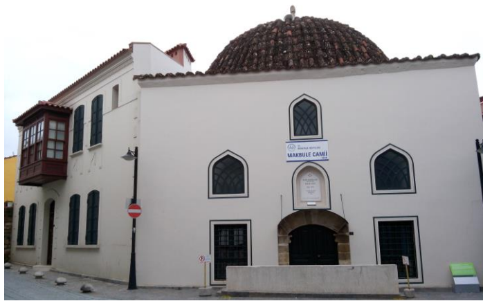
Figure 140 Northern Facade of the Makbule Kara Molla Masjid
