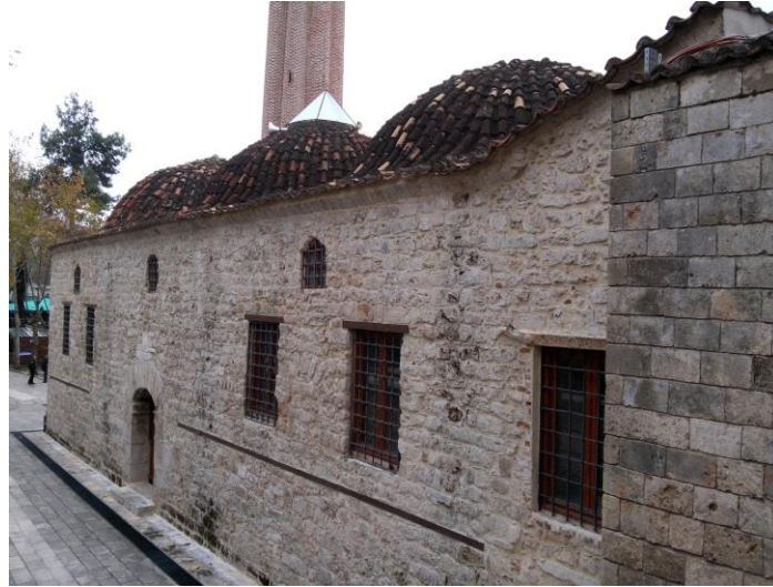
Figure 57 Northern Facade of the Yivli Minare Mosque Photograph by Melike Yılmaz
