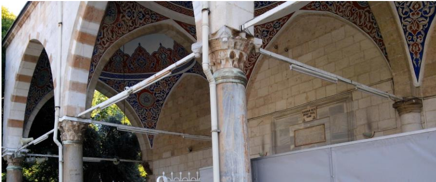
Figure 145 Roof of the the Murat Paşa Mosque's Narthex
