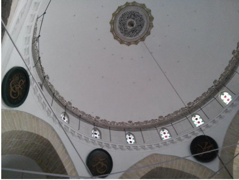
Figure 163 Dome of the Mehmet Paşa Mosque
