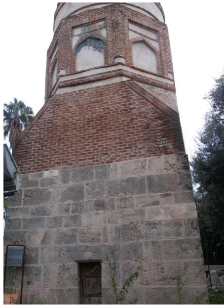
Figure 60 Northern Facade of the Yivli Minaret
