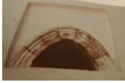
Figure 93 The Gap on the Western Wall of the Ahi Yusuf Tomb
