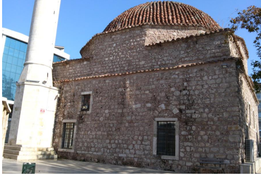
Figure 133 Western Facade of the Bali Bey Mosque
