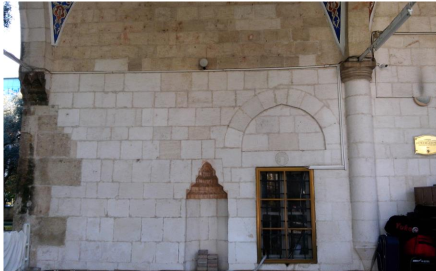
Figure 146 Eastern side of the Northern Wall of the Murat Paşa Mosque
