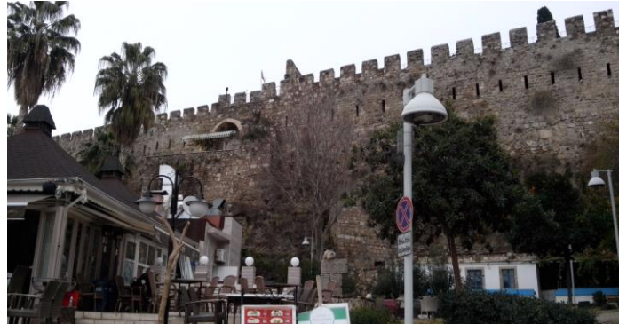
Figure 43 Middle Part of the Walls
