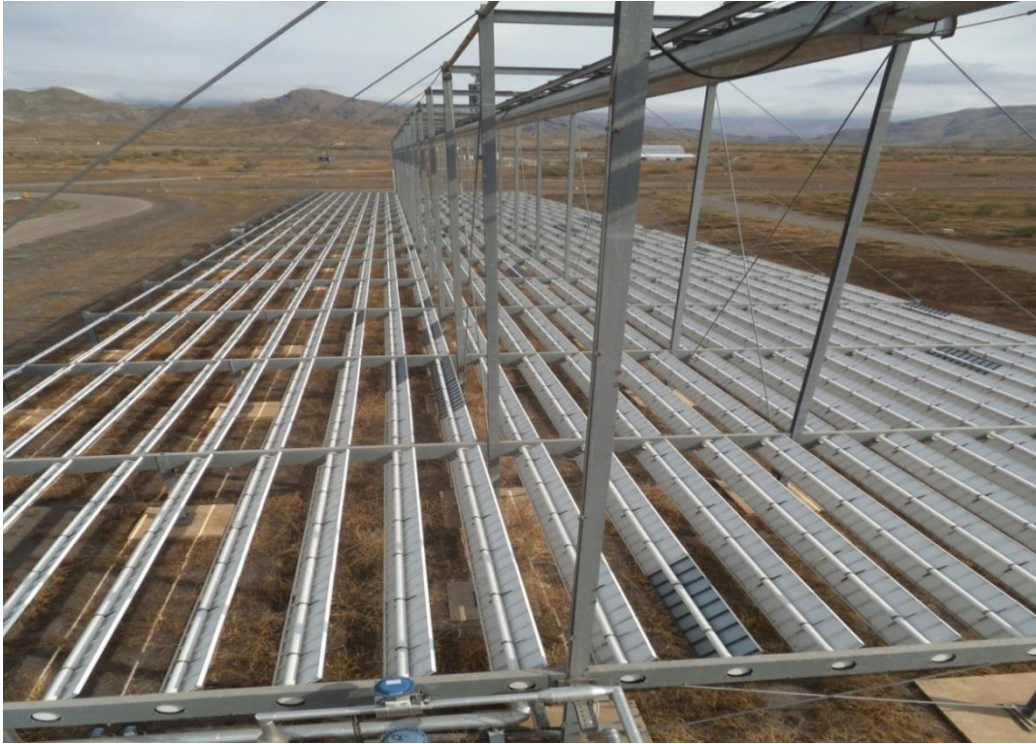
Figure 1.14 LF parked position at Plataforma Solar de Almería (PSA), Spain (Photographed by D.Baker and used with permission).
