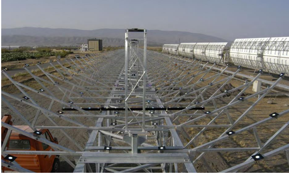
Figure 3.6 Space frame and mirror mounting points of a concentrating collector [46].
