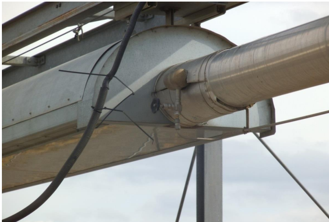
Figure 1.5 An installed LF receiver at Plataforma Solar de Almería (PSA), Spain (Photographed by D.Baker and used with permission).
