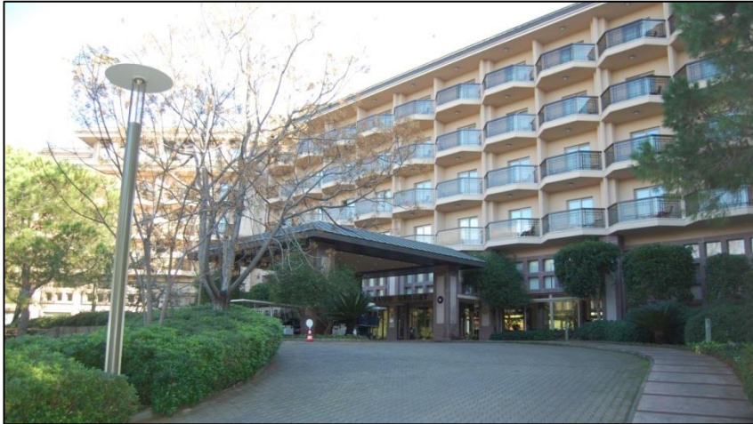
Figure 117 North-west elevation of the main building (taken by the author, December 2013).
