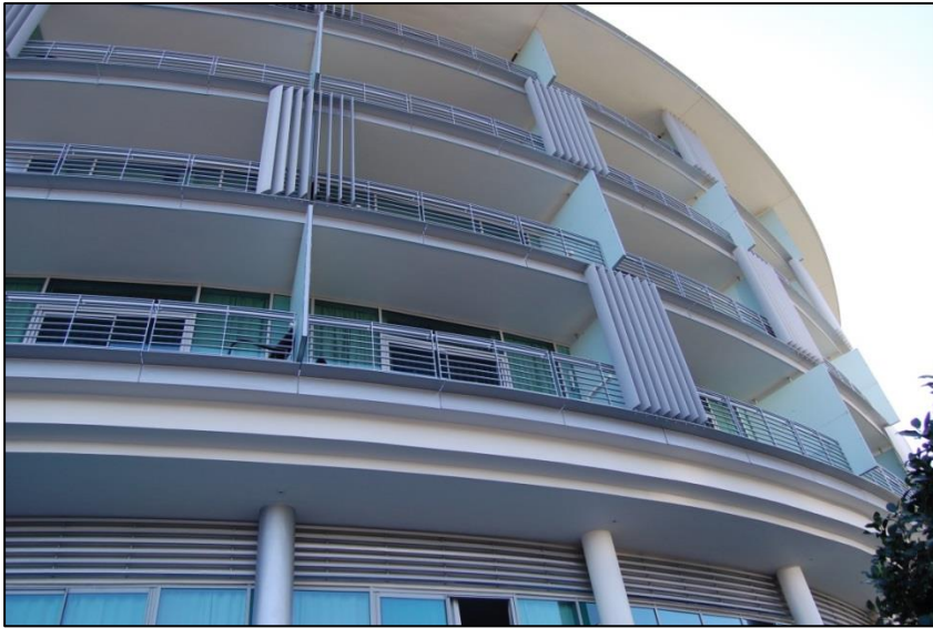
Figure 136 Facade of the main building (taken by the author, December 2013).
