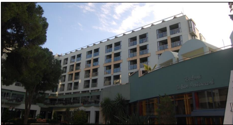
Figure 93 The northeast elevation of the main building (taken by the author, December 2013).
