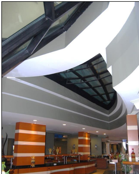
Figure 53 The toplight over the restaurant is covered with a plastic material (taken by the author, December 2013).
