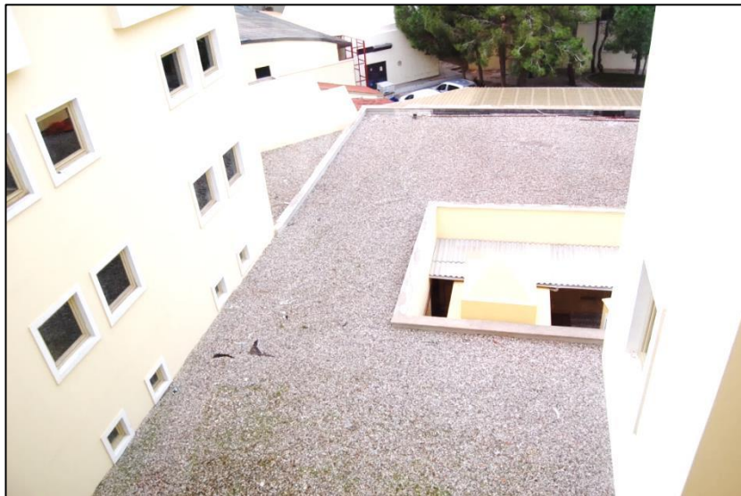
Figure 59 Flat roof (taken by the author, December 2013).
