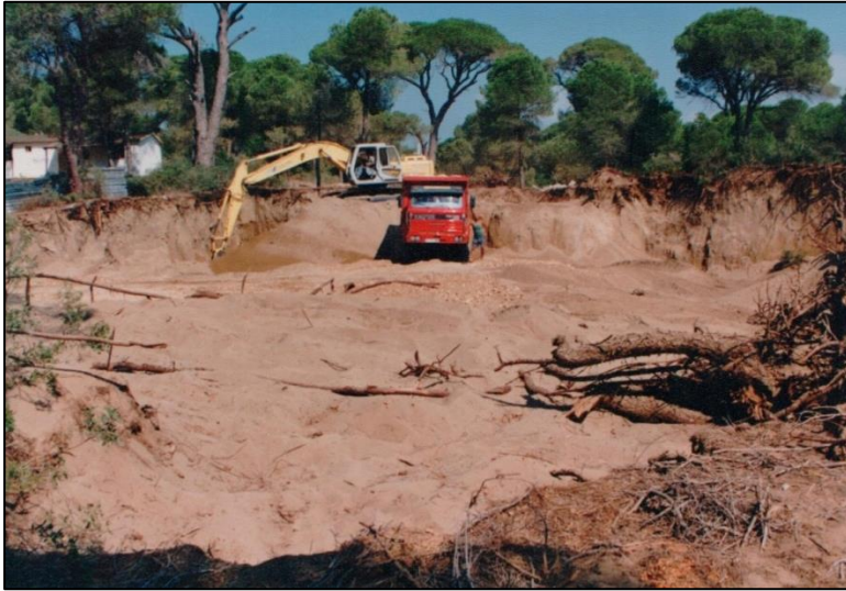
Figure 72 Excavation work (archieve of Ministry of Culture and Tourism).
