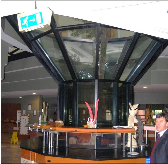
Figure 54 The toplight is arranged so as to protect an existing tree (taken by the author, December 2013).
