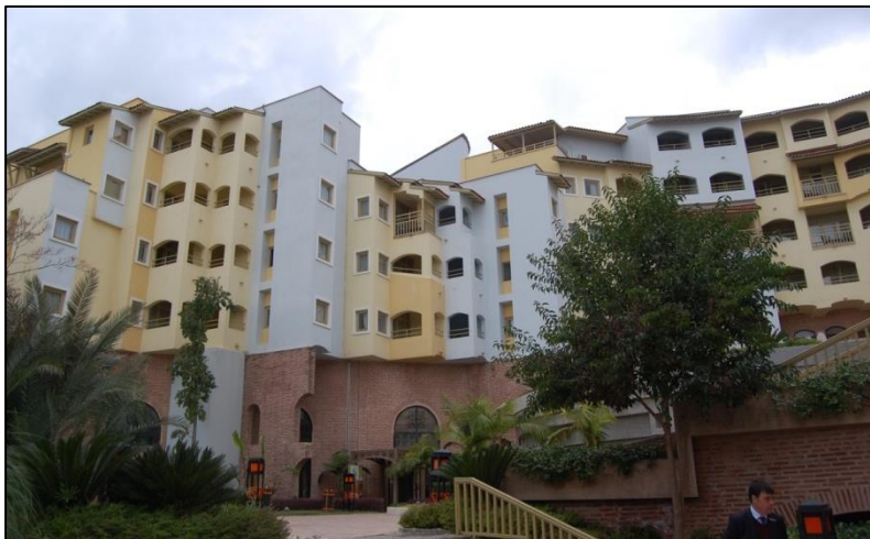
Figure 63 Various window types on the facades of the building (taken by the author, December 2013).
