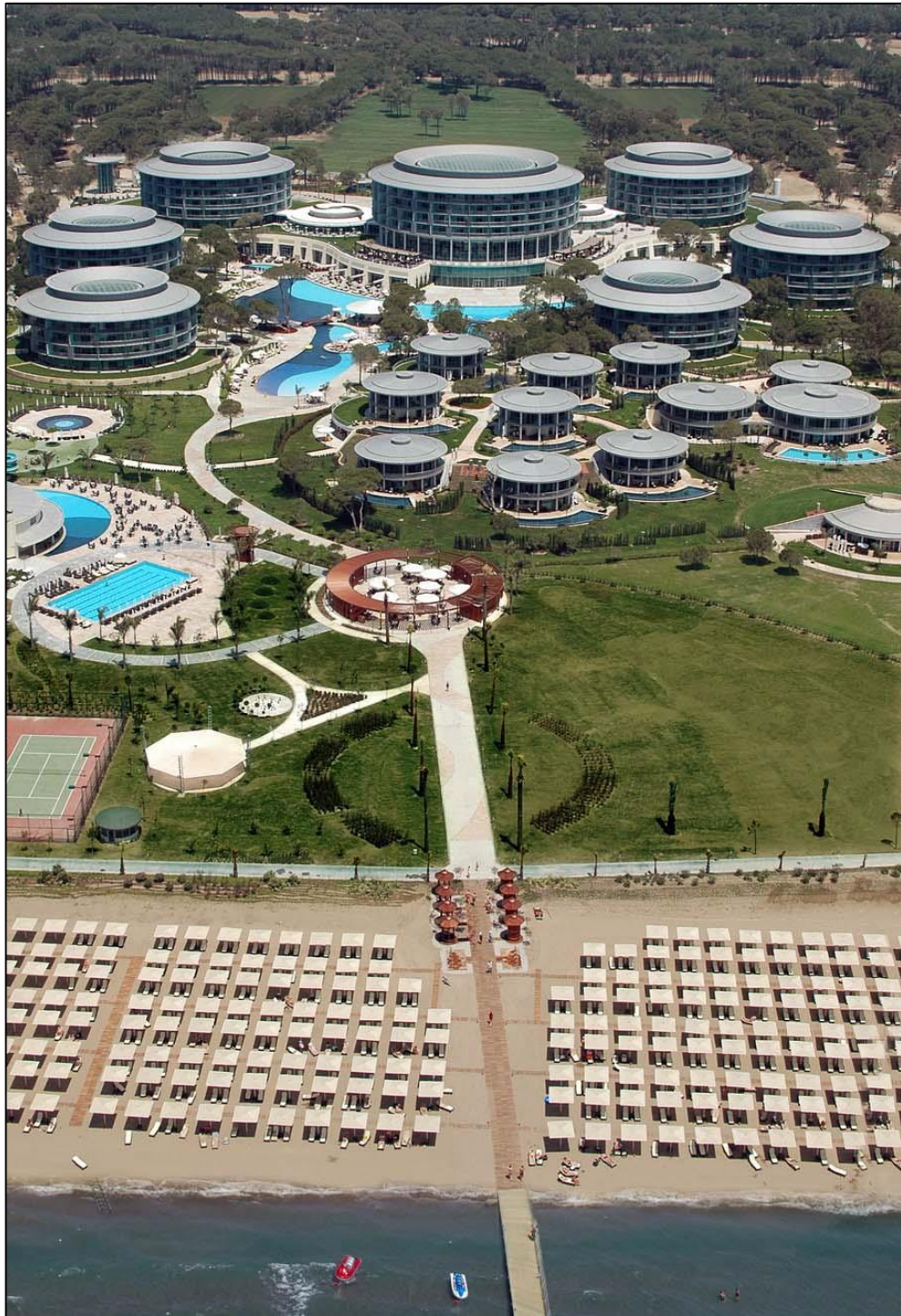
Figure 122 A general view of Calista Luxury Resort Hotel ( http://v3.arkitera.com/ , last visited on January 2014).
