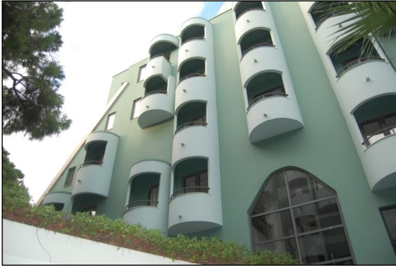
Figure 101 The balconies on the South elevation of the P Block (taken by the author, December 2013).
