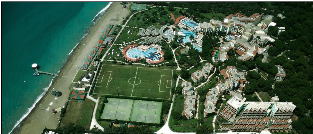
Figure 34 General view. ( http://limakhoteles.com/arcadia/download/ , last visited on March 2015)
