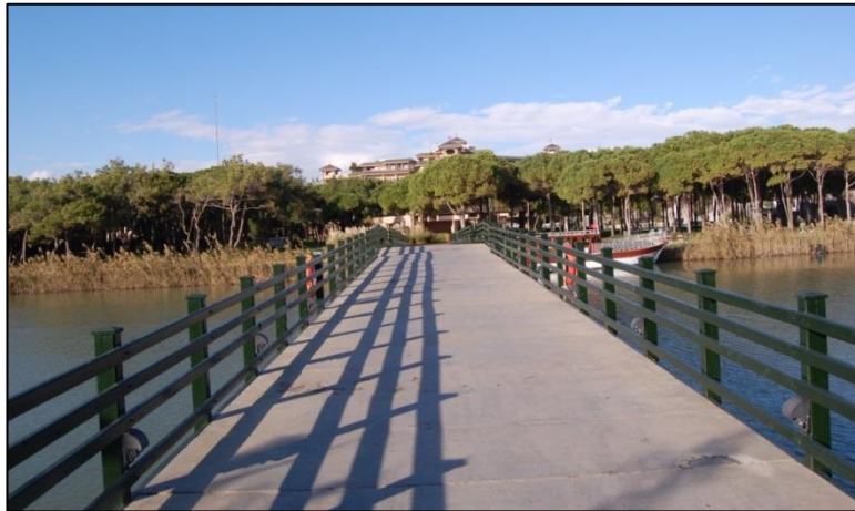
Figure 111 The view of south part of the land from the bridge (taken by the author, December 2013).
