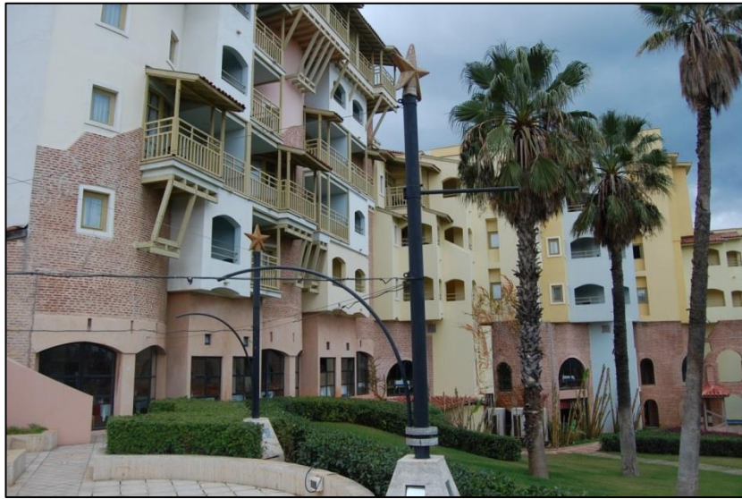
Figure 58 Exterior walls of the main building (taken by the author, December 2013).
