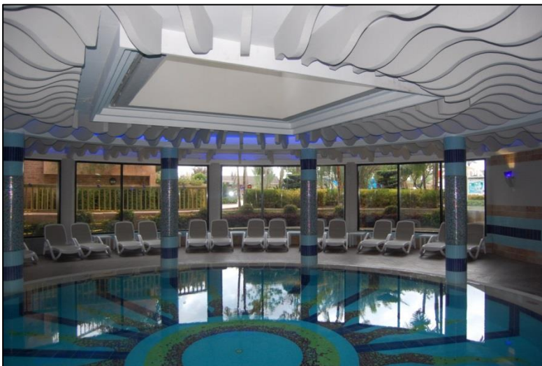
Figure 55 The sidelight and toplight fenestration in the swimming pool (taken by the author, December 2013).
