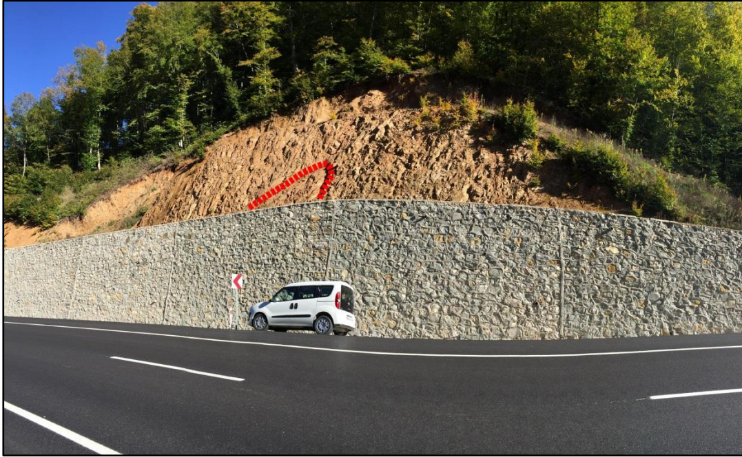
Figure 34. General view of the cut slope at Stop 4 (Failure zone indicated with red dashed line)
