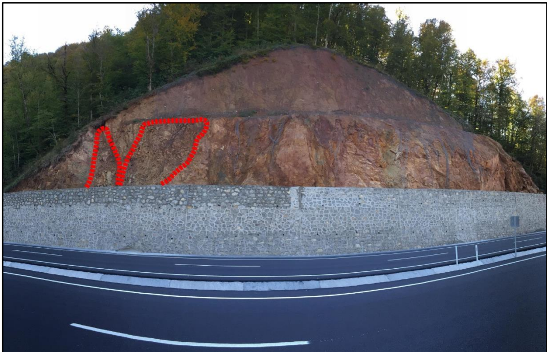
Figure 37. General view and shear zones of Stop 5 (Shear zones indicated with red dashed lines)
