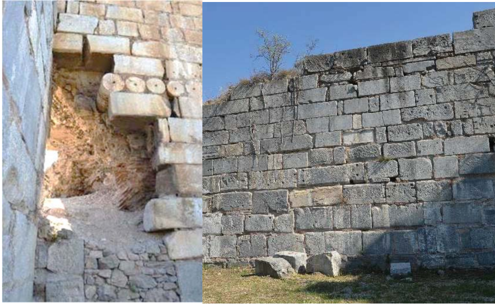
Figure 2-38: The core of the T70 (left) and the wall with stone masonry (right) (author, September 2015)
