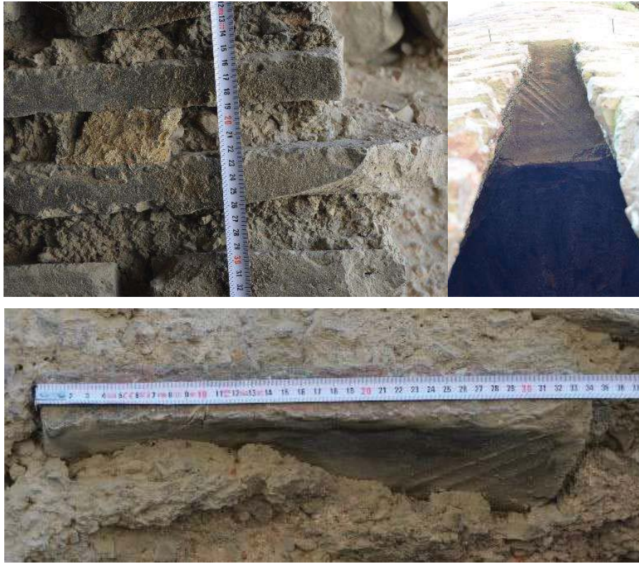
Figure 2-35: Dimensions of the brick and the finger marks on the brick (author, September 2015)
