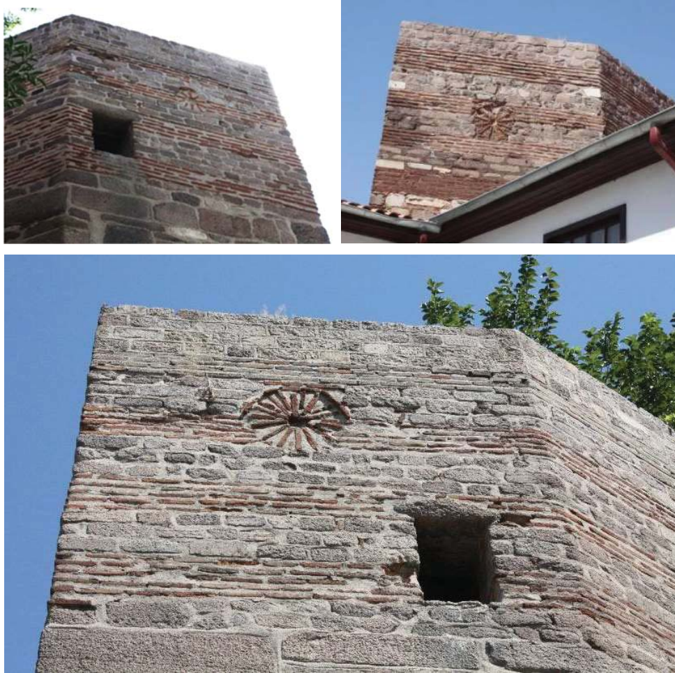
Figure 3-17: Alternating rows of brick and rubble stone with brick decoration typically of the Byzantine period (author, September 2016).
