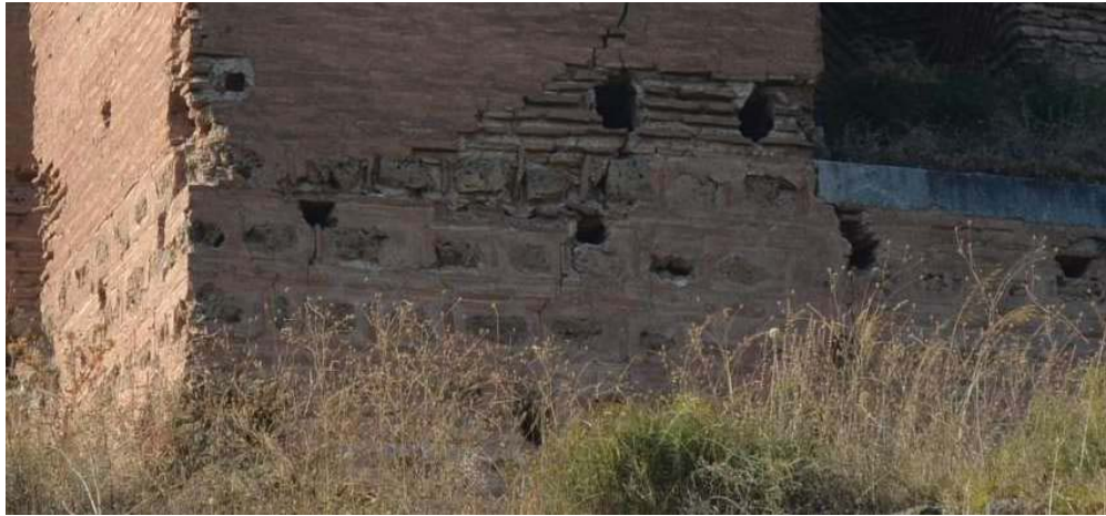
Figure 2-37: Cloisonné technique on Tower 106 (author, September 2015)
