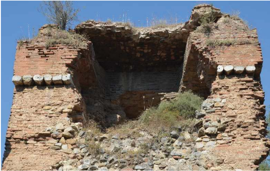
Figure 2-25: Superstructure of T66, showing the chamber with spolia (author, September 2015)
