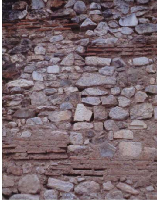
Figure 2-6: The southern facade of Iznik walls, traces of deformation (Adatepe and Arel, 2006)
