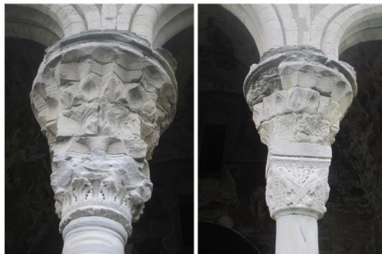
Figure 52 Two decked column capitals at the west facade. (Archive of Aysıl Tükel Yavuz, 2015).
