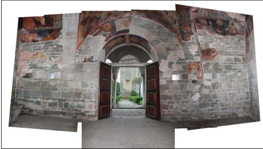
Figure 25 West wall of the Z2, 2014.
