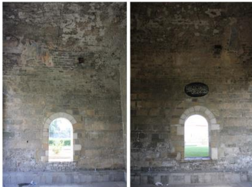
Figure 71 Openings at the east and west of the south porch (Z8), 2014.
