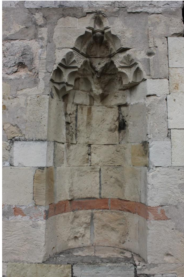
Figure 53 Niche with stalactites at the west façade, 2014.
