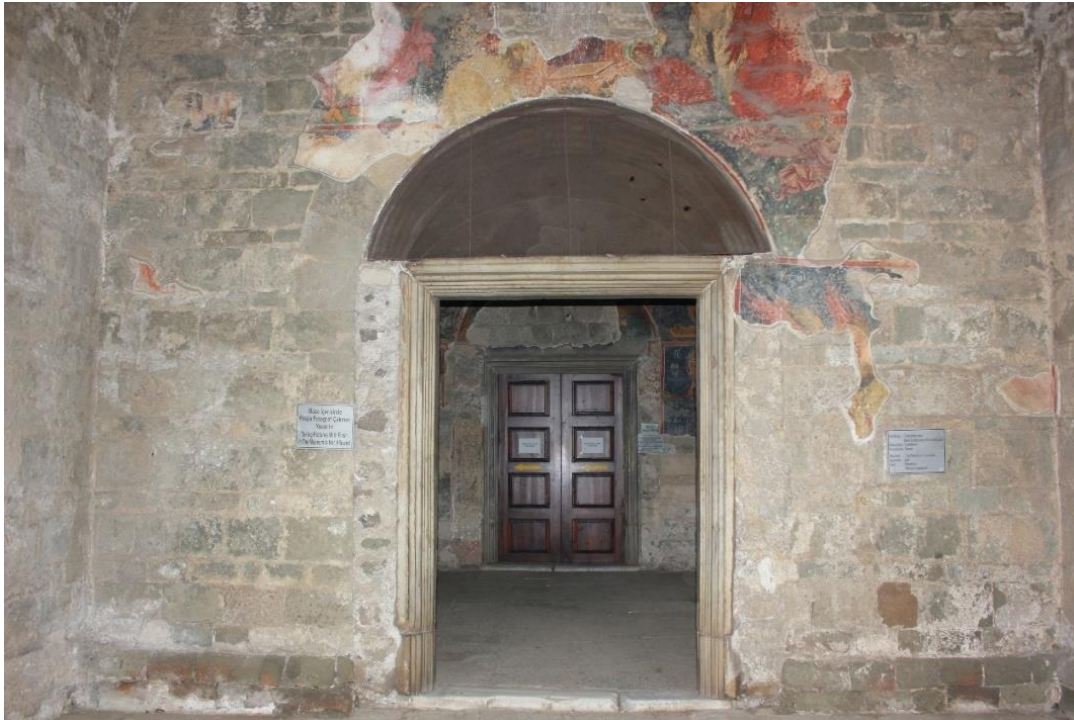
Figure 20 East wall of the Z1 space, 2014.
