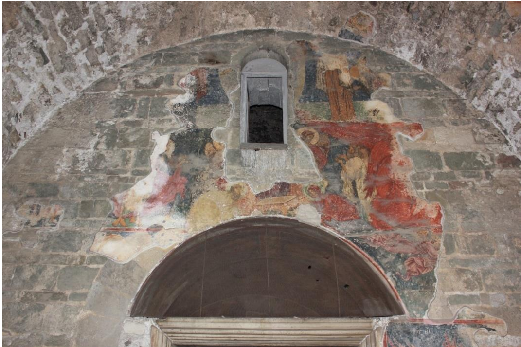
Figure 19 East wall of the Z1 space, 2014.
