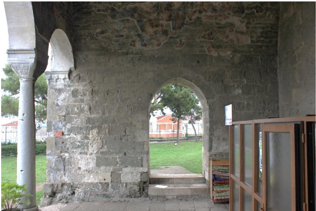
Figure 37 East wall of the Z7 Space, 2014.
