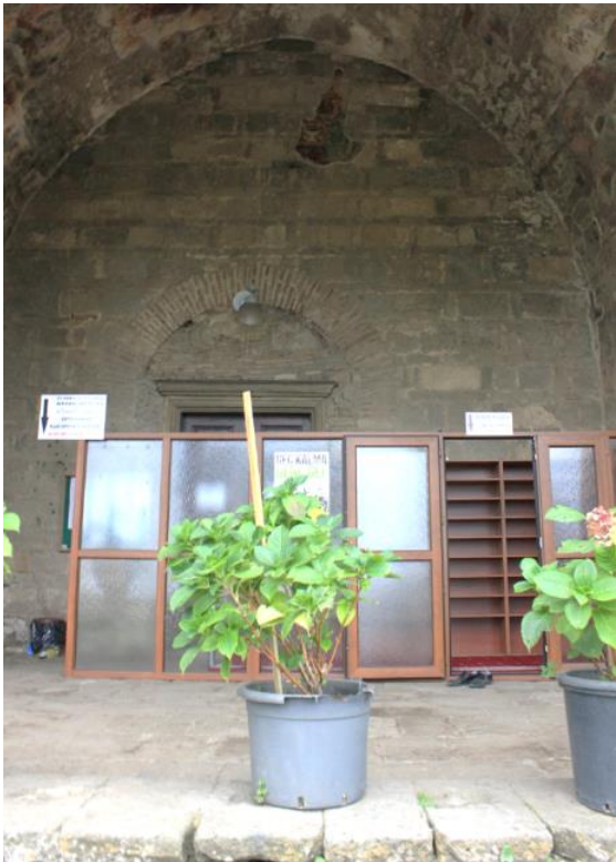
Figure 39 Entrance to the Z3 space at the south Wall of the Z7 Space, 2014.
