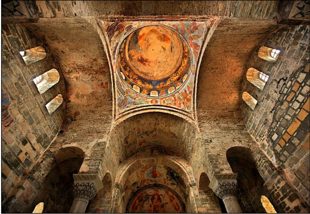
Figure 31 View of the dome from interior (Archive of Pious Foundations Directorate of Trabzon).
