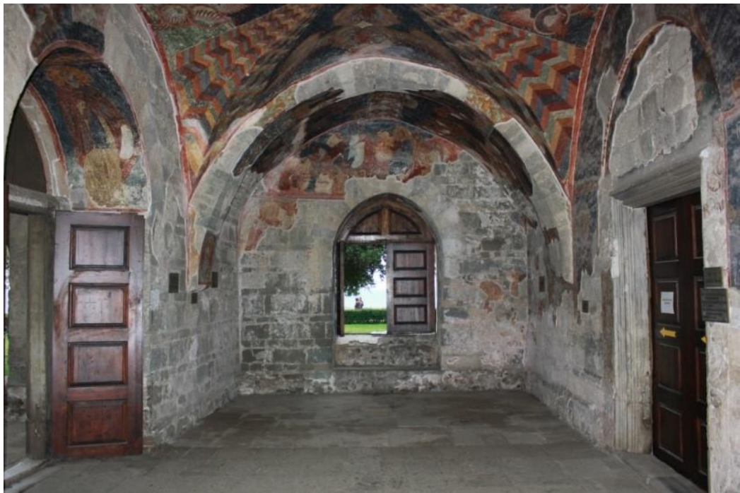
Figure 22 North wall of the Z2, 2014.
