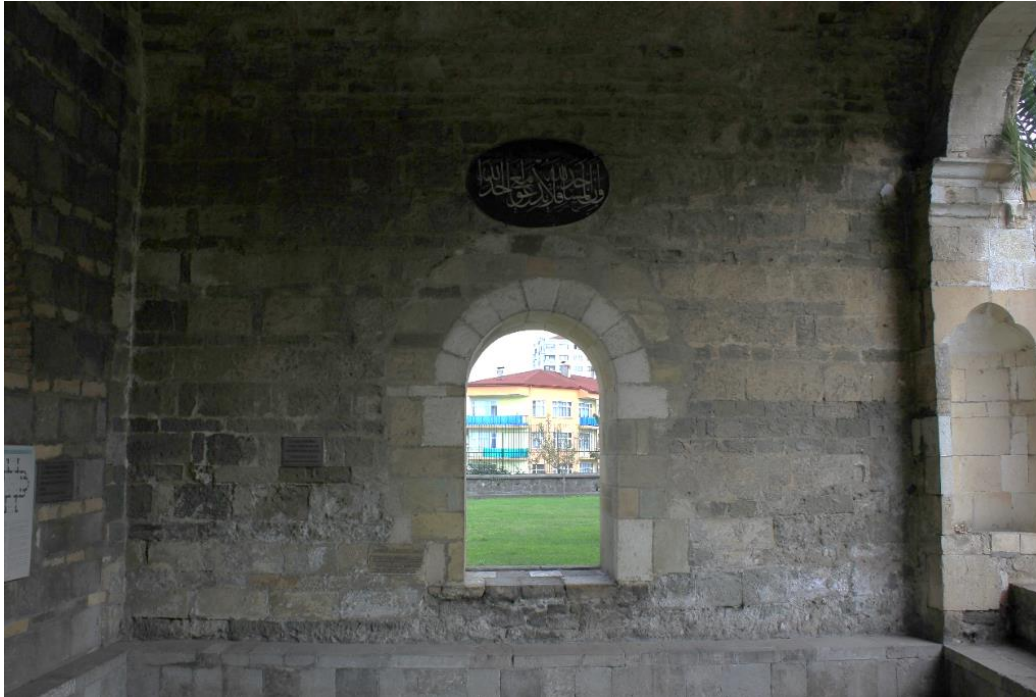
Figure 42 East wall of the Z8 space, 2014.
