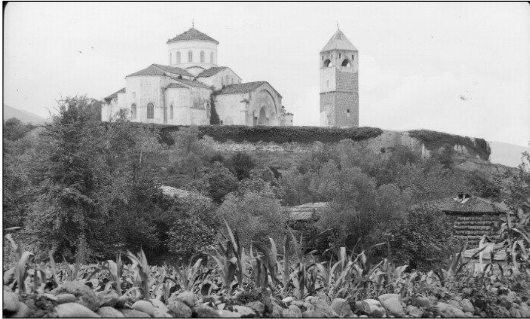
Figure 12 Old photo of the Hagia Sophia from north-east, 1960's before the restoration. (Archive of Pious Foundations Directorate of Trabzon).
