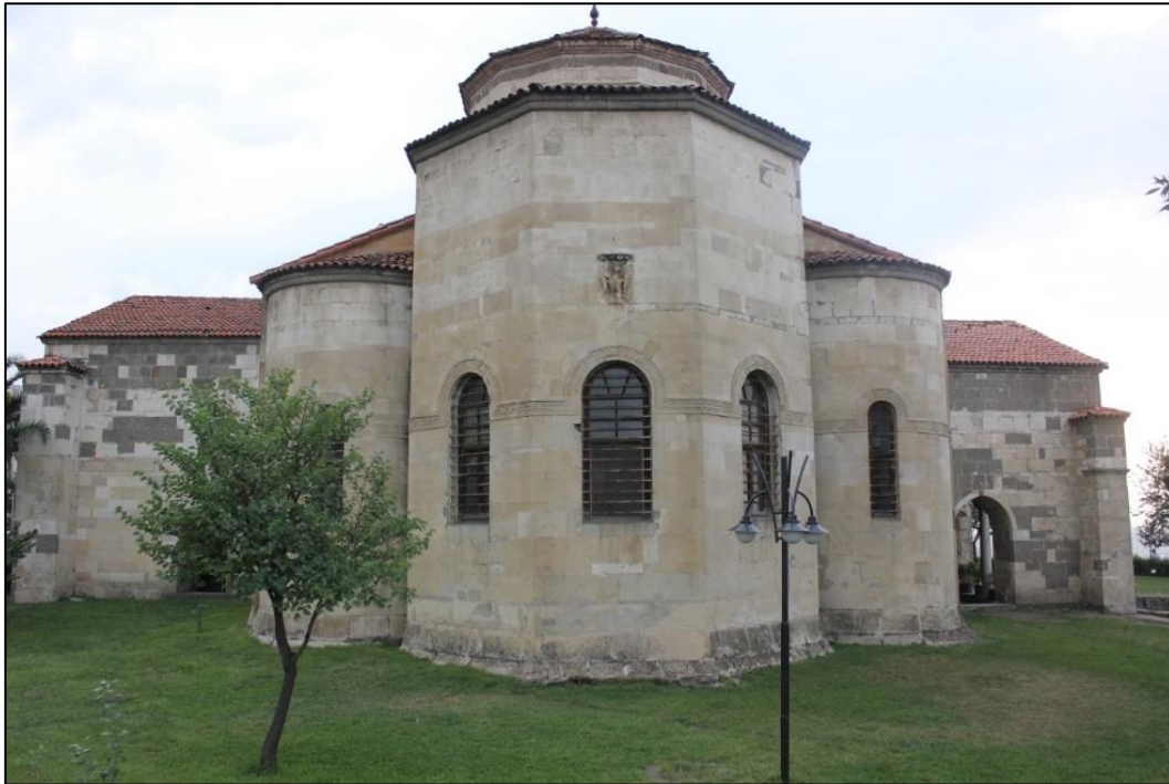
Figure 45 East Façade, Exterior of Apses, 2014 (Z4, Z5, Z6).
