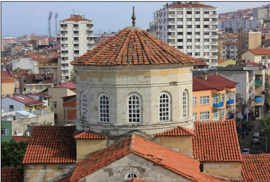
Figure 32 View of the dome from the west, 2014.
