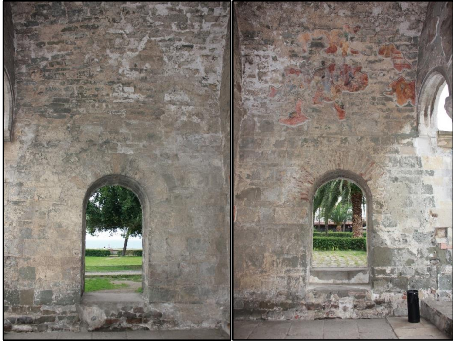
Figure 18 North and south walls of the Z1 space, 2014.
