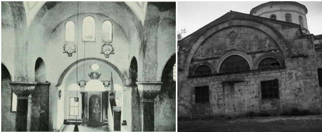
Figure 70 South wall of the naos and south porch before the Edinburg University Restoration. (Archive of Pious Foundations Directorate of Trabzon).
