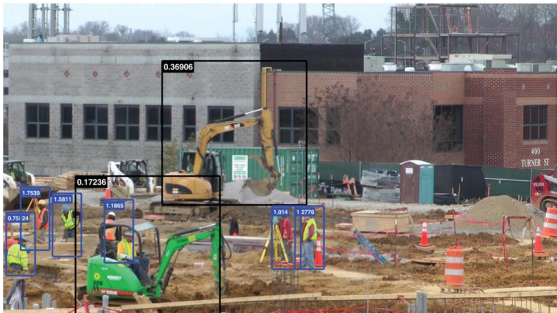
Figure 1 - Detection of Construction Equipment and Workers from Video Frames (Memarzadeh et al. 2013).
