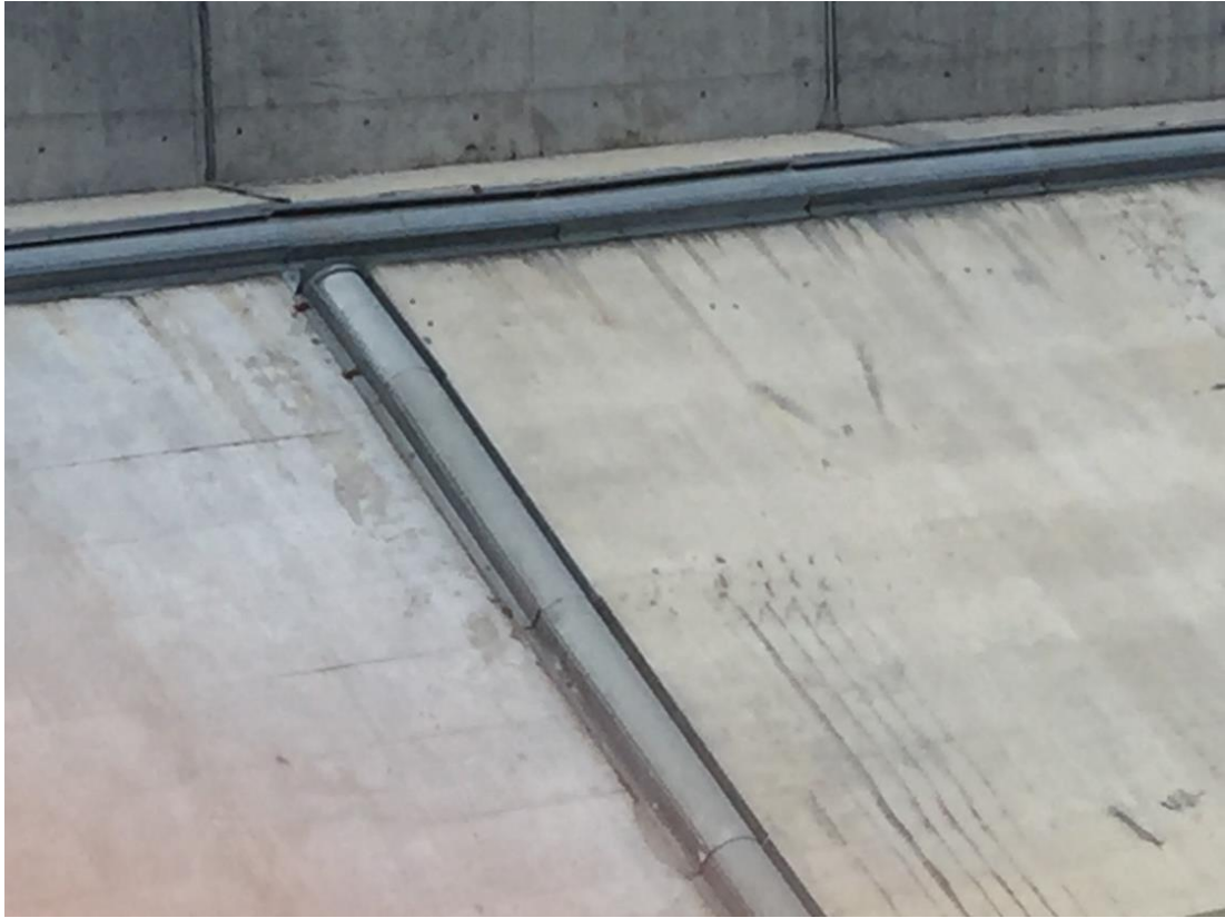
Figure 2.4 Close-up view of the face slab of Kavşak Bendi Dam
