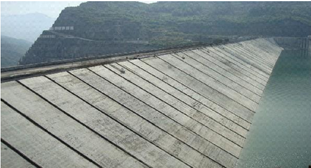
Figure 2.3 Concrete face slab of Shuibuya Dam (Materon, 2013)
