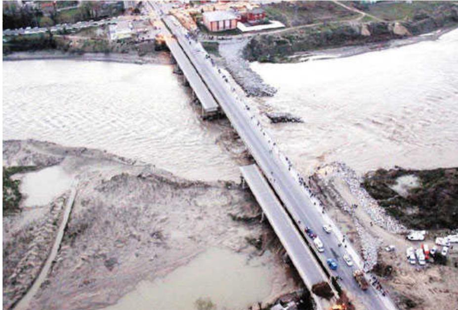
Figure 1.4. Collapsed view of Çaycuma Bridge after flood in 2012 (Sondevir, 2012)
