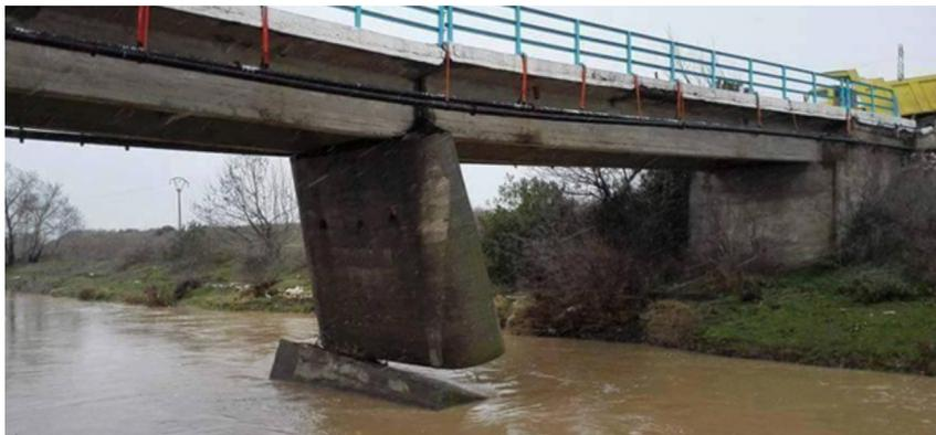
Figure 1.1. Yayakent Bridge view after flood in January, 2016 (Tuna, 2016)
