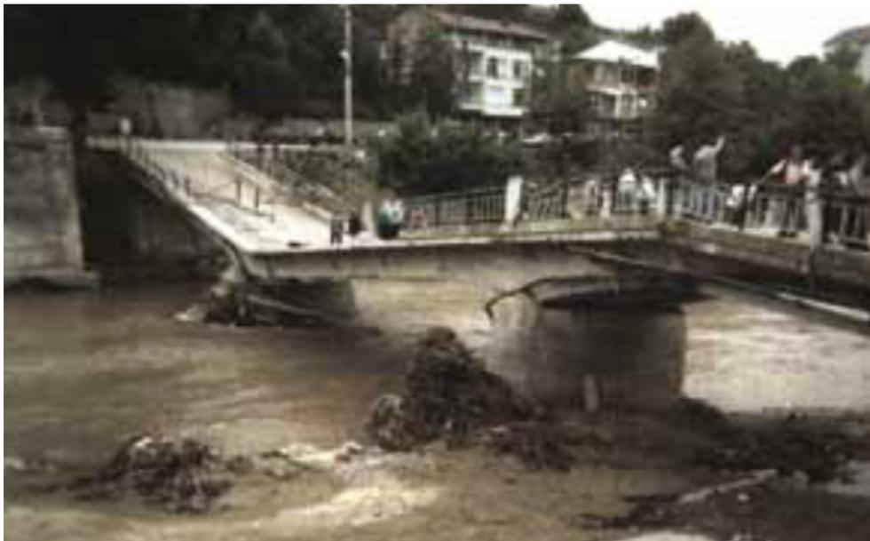
Figure 1.5. Damaged view of the bridge at Devrek due to scour (Yanmaz, 2002)
