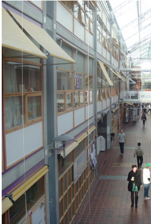
Figure 2.46: Different Glazing Area for Different Floors to Control the Natural Lighting, Trondheim, Norwegian University of Science and Technology, Campus Source: https://soraj.files.wordpress.com/2008/10/dsc
