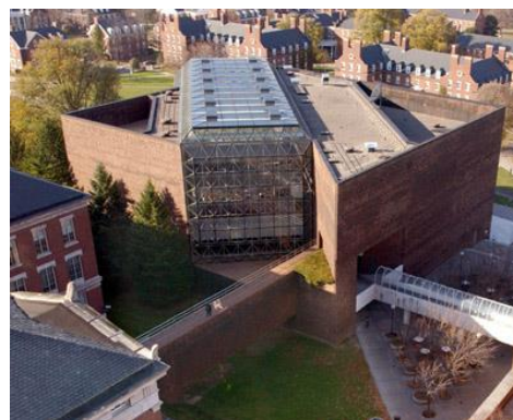
Figure 2.22: An Example of a Linear Atrium, University of Rochester, Wilson Commons Building Source: http://www.himberassociates.com/educat
