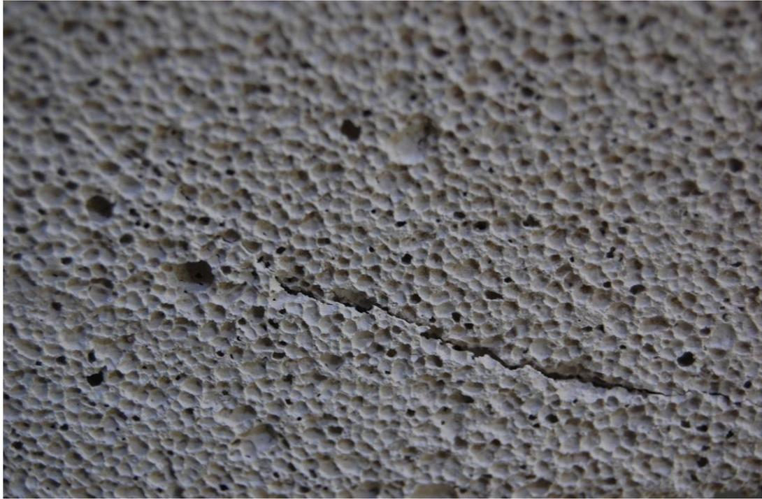
**Figure 4.24.** The macro view of the crack G2-g on the exposed G4 type AAC block (See in reference to Figure 4.17).
