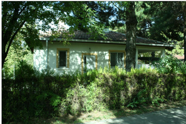
exterior view from south
