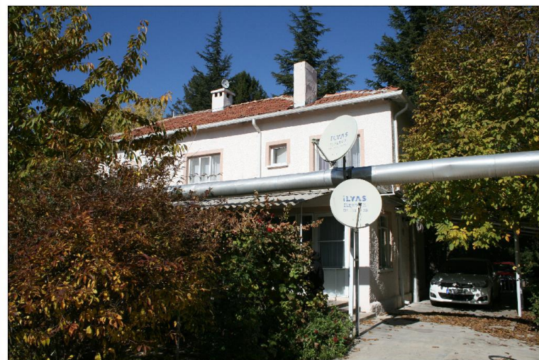
exterior view from south-east
