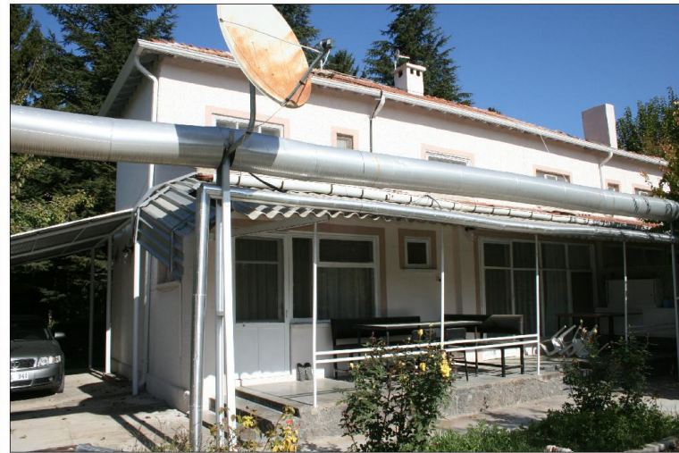
exterior view from south-west
