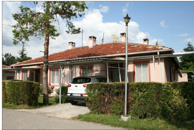
exterior view from south-west
