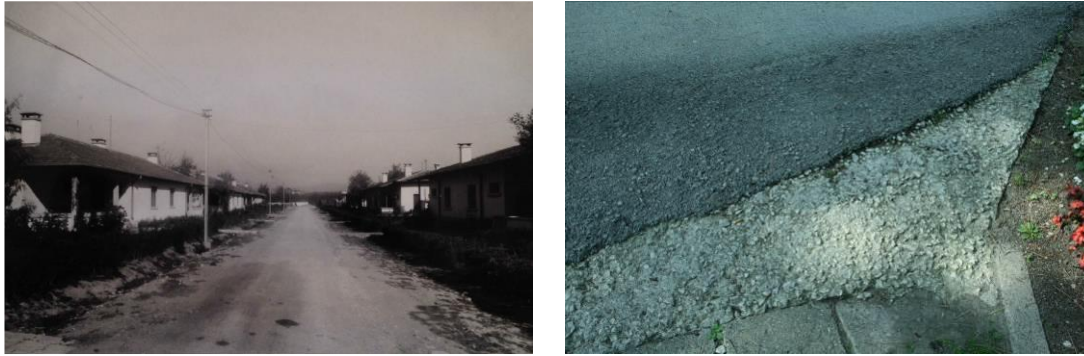
Figure 3.114: Original compact earth pavement and rough concrete pavement layers
