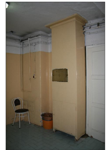
boiler in laundry room
