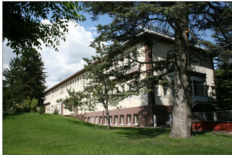
exterior view from south-west
