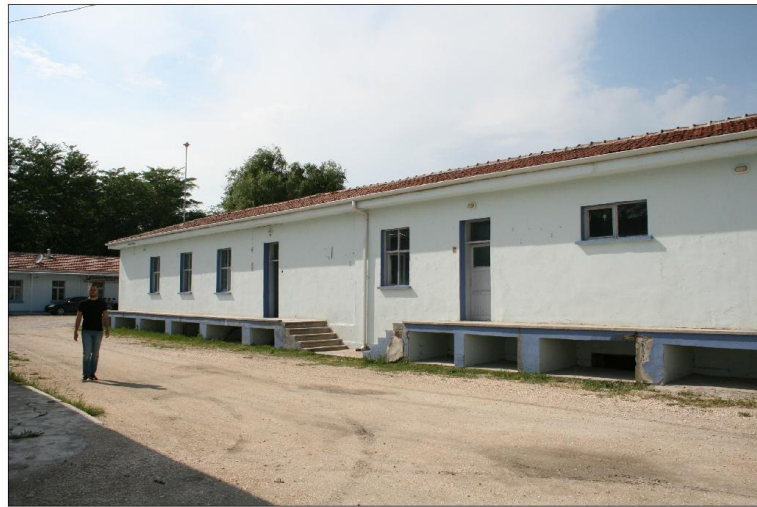
exterior view from north-east
