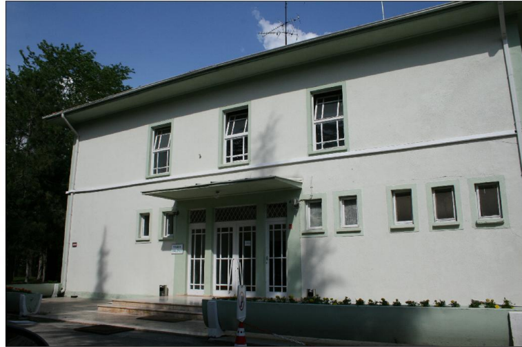
exterior view from south-west
