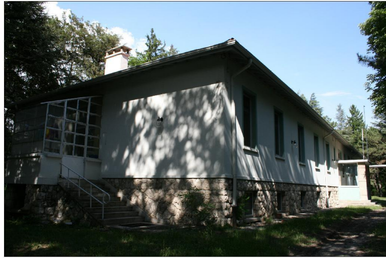
exterior view from north-west
