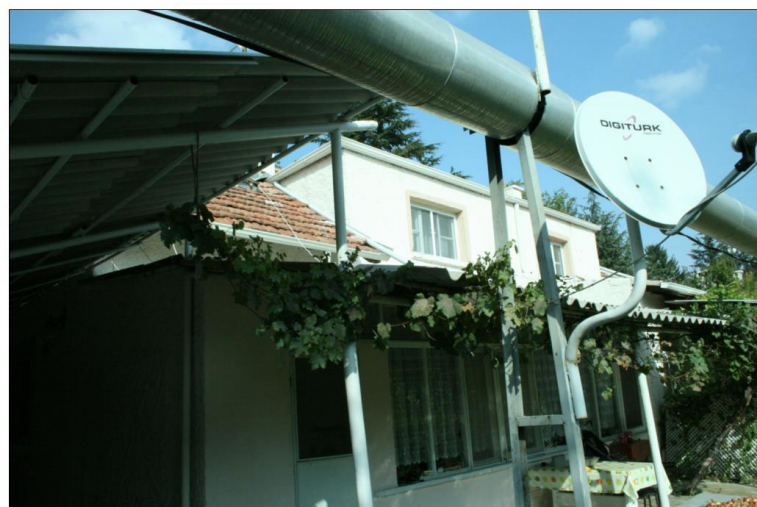
exterior view from south-west- additional mass
