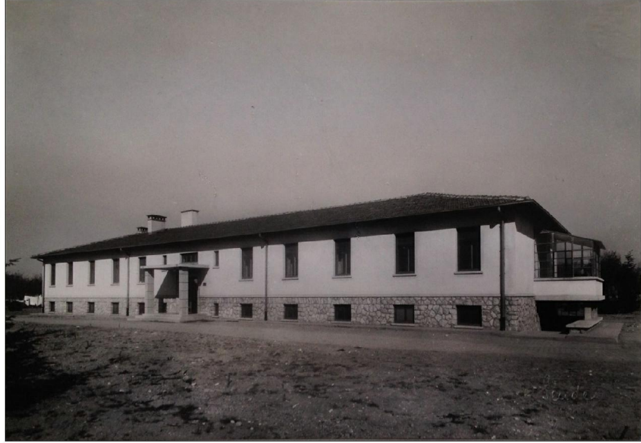
photo of Girl's Dormitory (Hospital, B13) front façade, 1949 courtesy of Eskişehir Sugar Factory Archives
