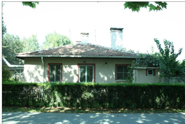
exterior view from north and wet space addition
