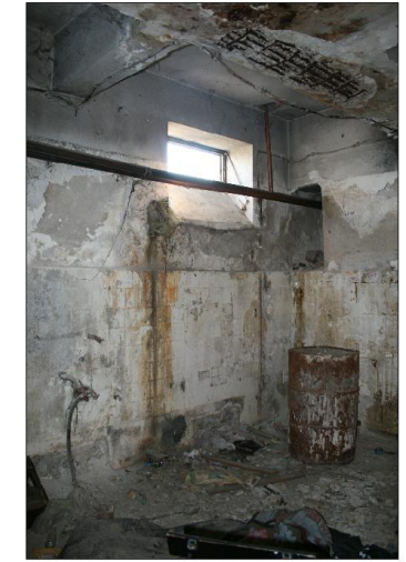
basement engine room window
