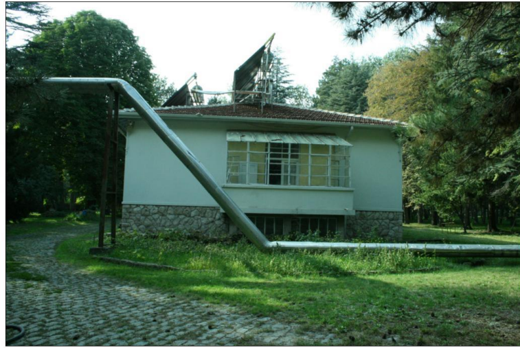
exterior view from south
