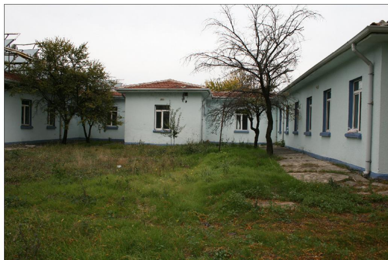
exterior view from south
