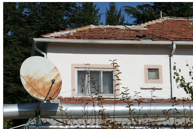
first floor windows
