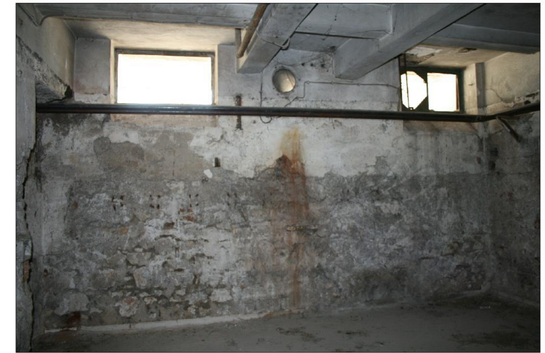
basement service room
