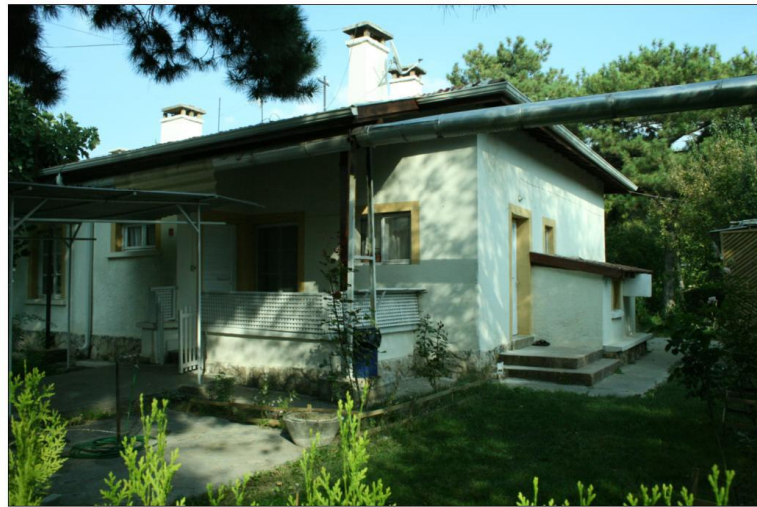
exterior view from south-west
