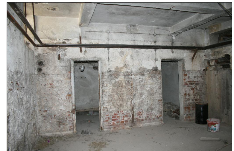
basement storage doors in service room
