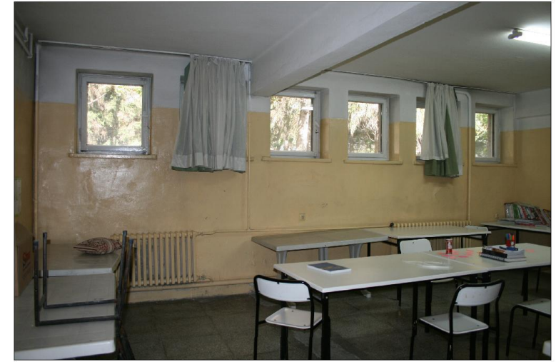
basement study hall
