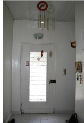
entrance door from inside
