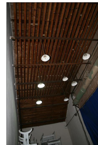
ceiling of stage
