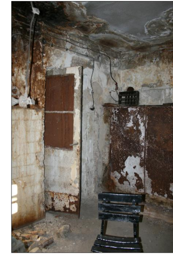
basement engine room door
