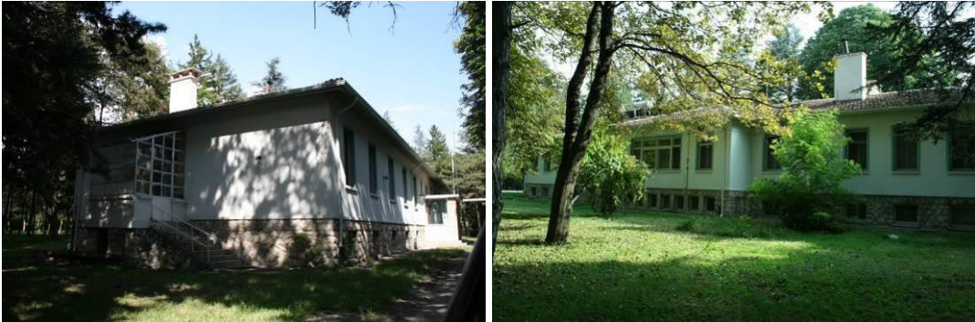
Figure 3.69: South-west and north façades of Girl’s Dormitory
