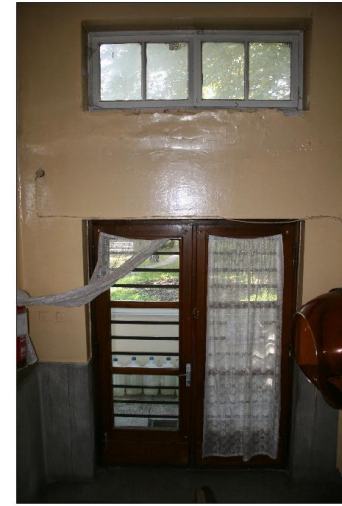
entrance door from inside
