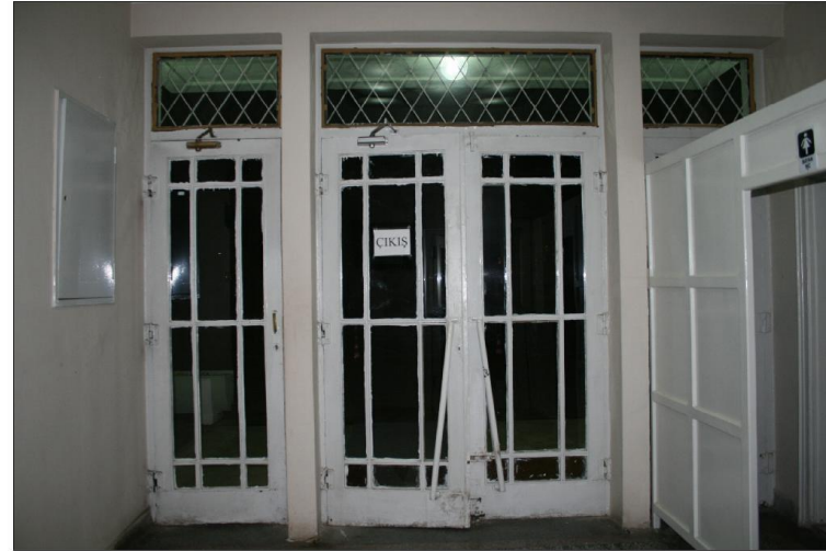
entrance door from inside
