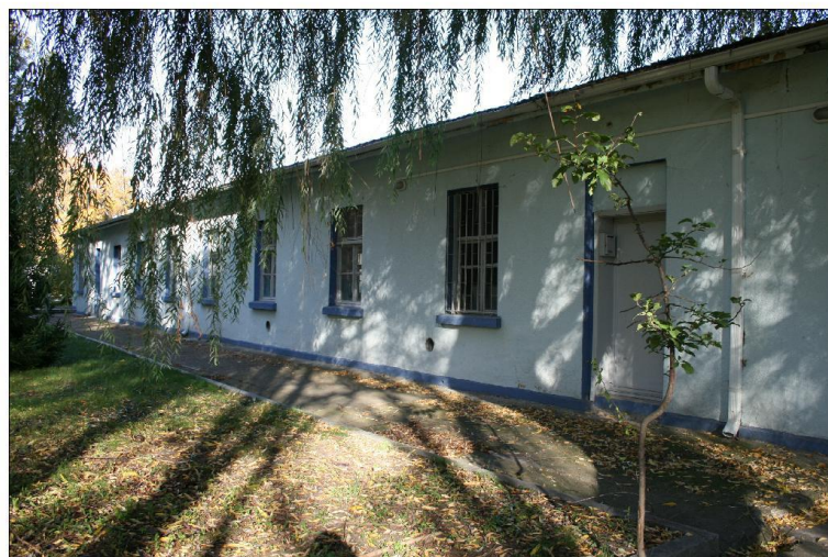
exterior view from south-west and altered opening
