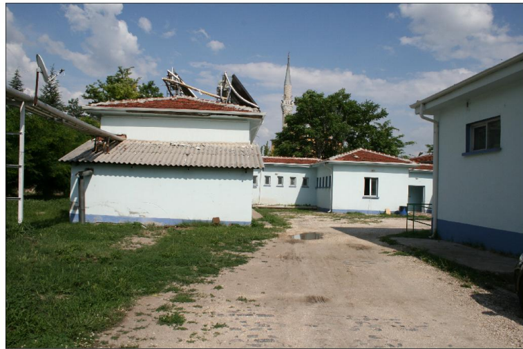
exterior view from west and mass addition
