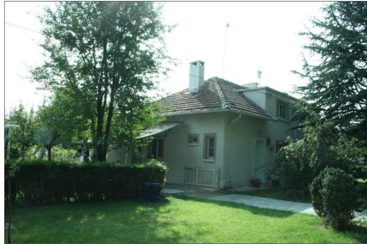
exterior view from north-east
