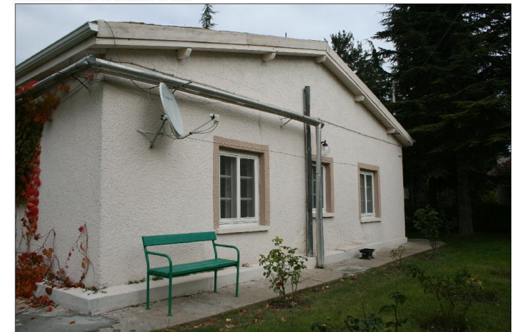
exterior view from south-west
