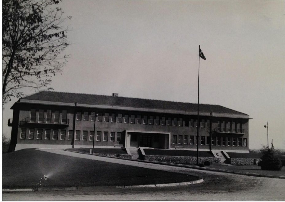
photo of front façade, 1949 courtesy of Eskişehir Sugar Factory Archives
