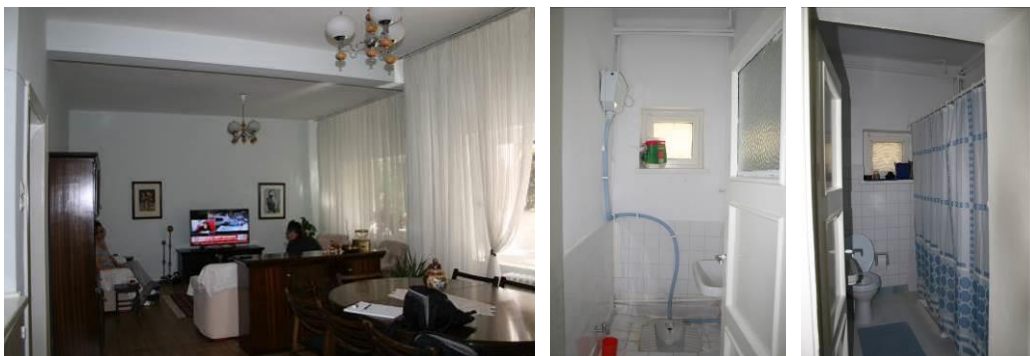
Figure 3.42: Examples of removal and alterations in Employee Dwelling Type 5
