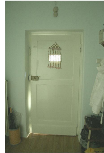
main entrance door from inside
