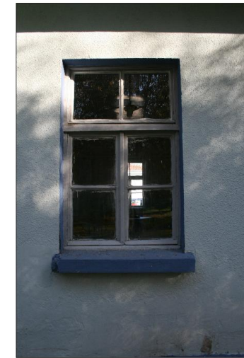
window from outside
