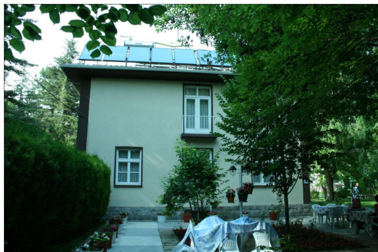
exterior view from south
