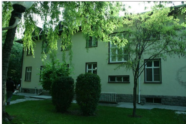
exterior view from north-east
