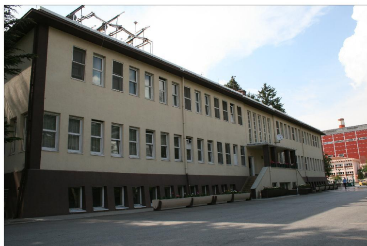
exterior view from south-east
