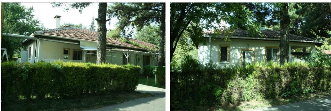
Figure 3.49: South-east and south façades of Employee Dwelling Type 7
