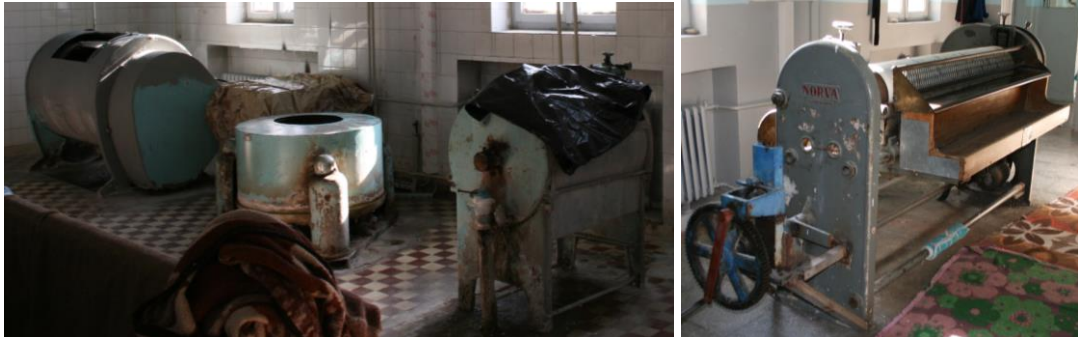
Figure 3.90: Original equipment of the Laundry that is still in-service
