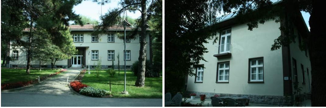
Figure 3.61: West and south façades of Old Guesthouse
