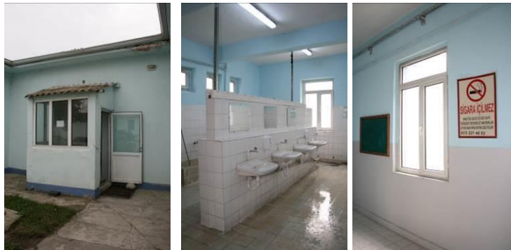
Figure 3.74: Examples of alterations in Worker's Pavilion
