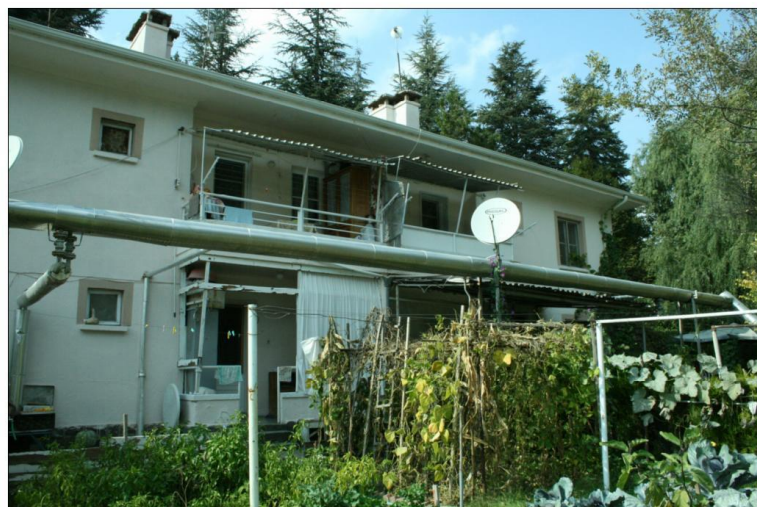
exterior view from south-east
