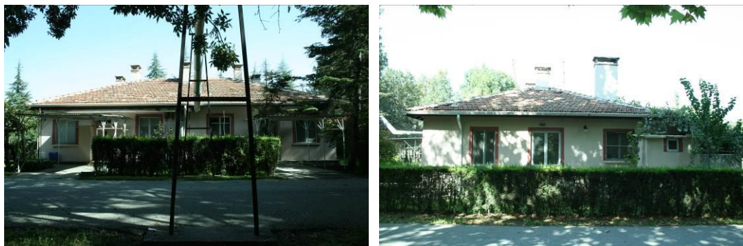
3.53: West and south façades of Employee Dwelling Type 8
