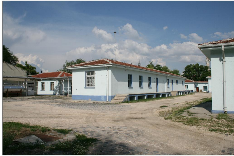
exterior view from south-east
