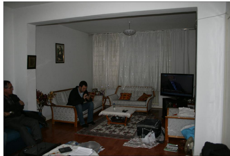
removal of wall
