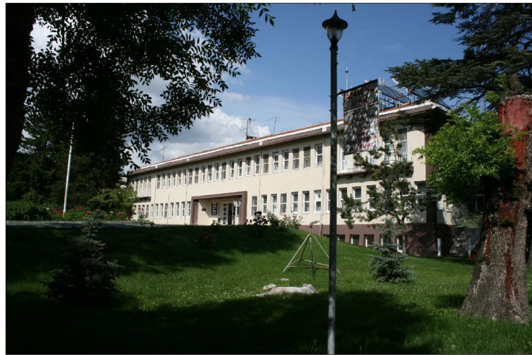
exterior view from south-west
