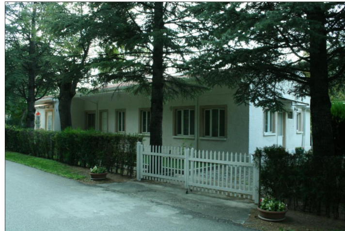
exterior view from north-east
