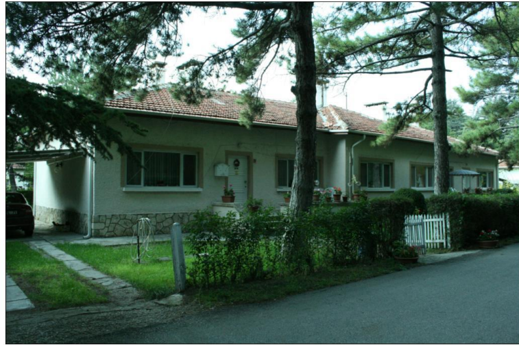
exterior view from south-east
