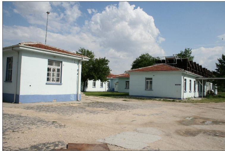
exterior view from north-west
