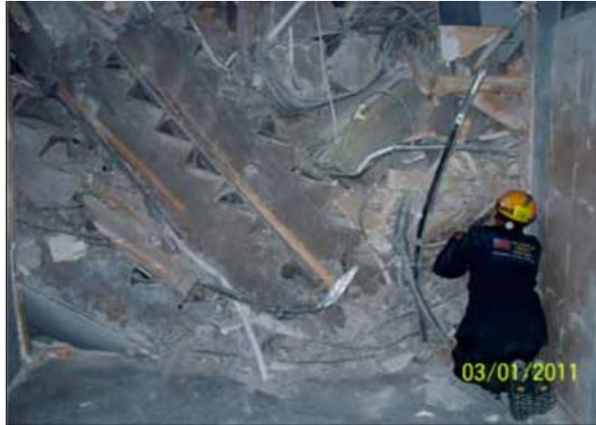
Figure 1-16: Collapsed Precast Concrete Stair in Multi-Story Building (Elwood, 2013)
