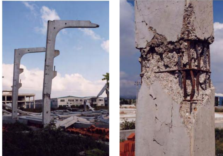
Figure 1-10: Severe Distress in Precast Concrete Column (FIB, 2003)
