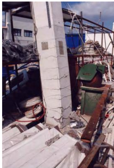
Figure 1-9: Ductile Flexural Yielding at a Precast Column (FIB, 2003)
