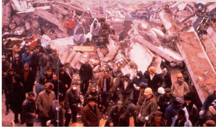
Figure 1-6: Collapse of Precast Buildings in Armenian Earthquake (Wyllie, 1989)
