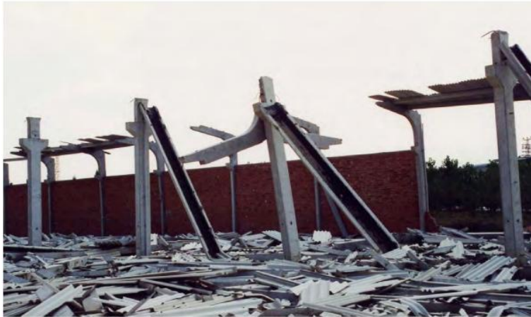
Figure 1-12: Failure of Cantilever Head Connection on Top of Columns (FIB, 2003)
