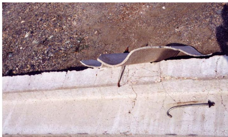
Figure 1-11: Flexible Connection Between Diaphragm and Precast Concrete Beam (FIB, 2003)
