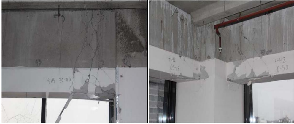
Figure 1-14: PWC Tower precast moment frame damage (Fleischman, 2014)
