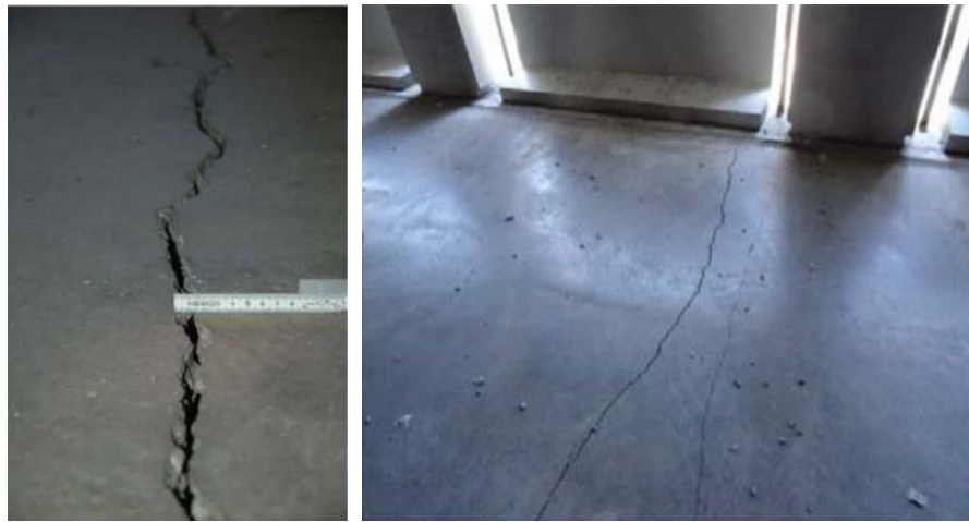
Figure 1-15: Damage in Floor System in Brannigans Tower (Fleischman, 2014)
