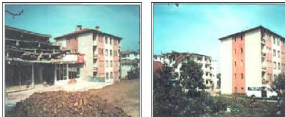
Figure 1-7: A Precast Concrete Building with no Damage after Kocaeli Earthquake, 1999 (Ghosh, 2001)
