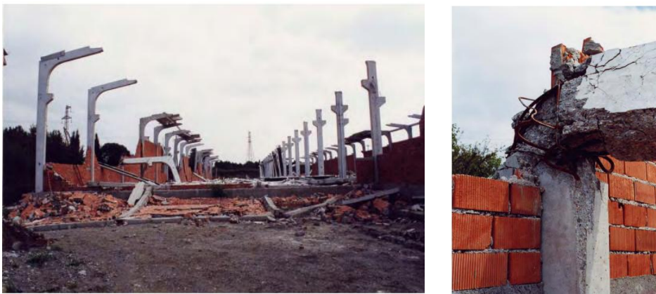
Figure 1-13: Failure of Columns due to Interaction with Stiff Masonry Infills (FIB, 2003)
