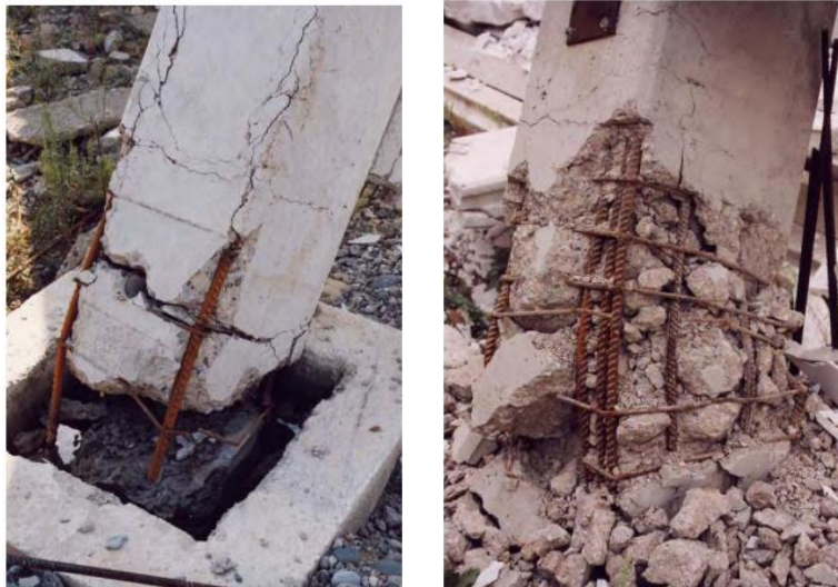
Figure 1-8: Shear Failure of Precast Concrete Column (FIB, 2003)
